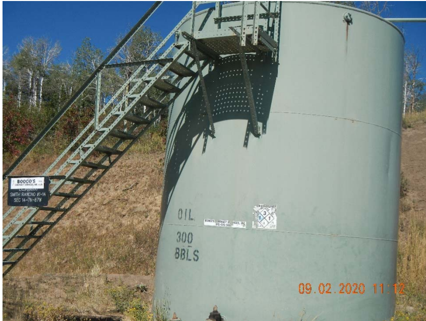
Photo 4. Tank labels faded and peeling.
