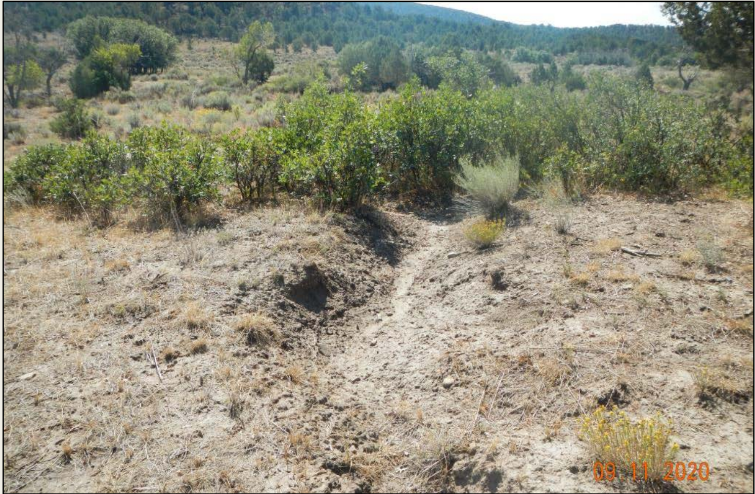
Photo 3. View of erosional channel, approximately two feet wide and deep, forming from a shallow headcut in the southwestern corner of the project area.
