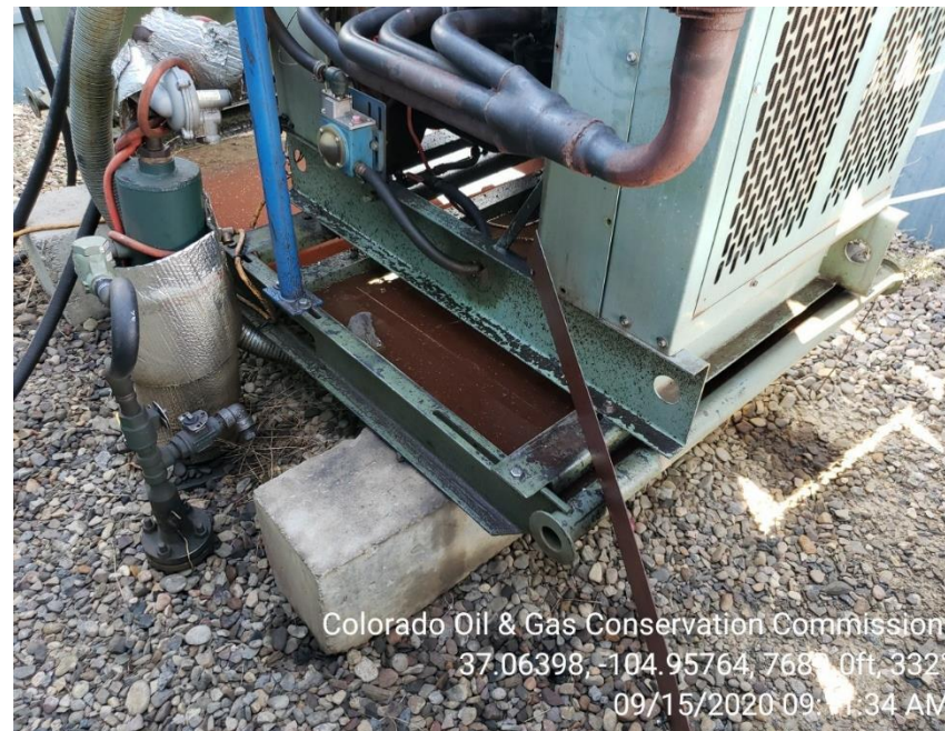
Photo 4 Stained soil at engine skid
