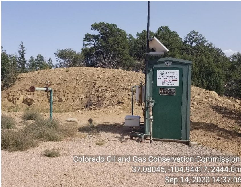
Photo 1 location sign. Risers not LOTO unused equipment separator house due to well being TA
