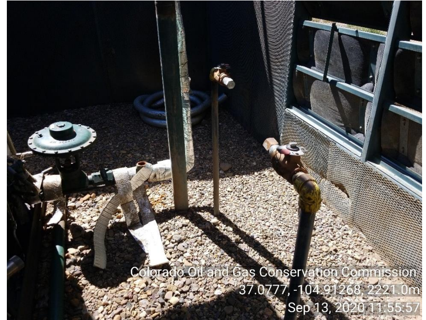
Photo 10 1" risers in liquid ring sound walls not LOTO
