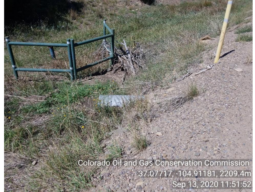
Photo 6 culvert in pic 5 is plugged on outlet side in creek
