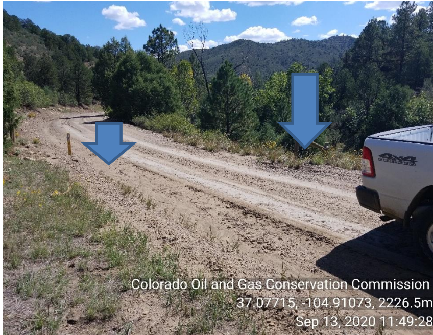
Photo 3 road between Big bingham entrance and AC 17-14 not properly maintained bar ditch full of sediment causing storm water to cross road and go into Big Bingham water way
