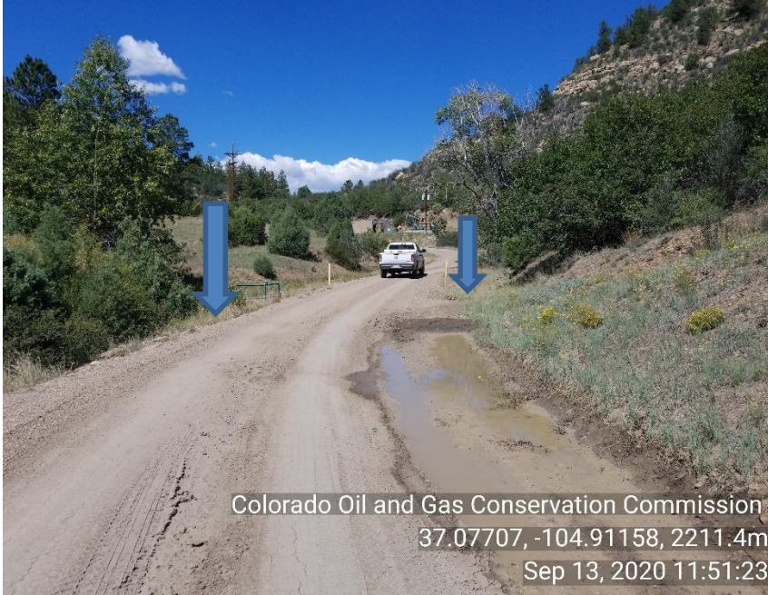
Photo 5 Road between big Bingham entrance and AC 17-14 not properly maintained. Drainage from hillside causing sediment to build up on road way.
