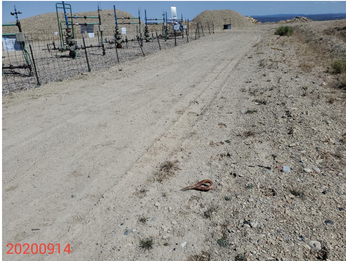
Photo 5: Photo shows example of guy line anchors observed on the Location without proper markers pursuant to Rule 1003.a
