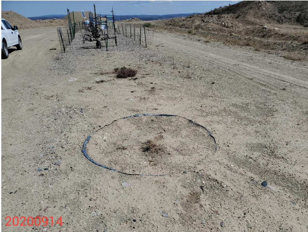
Photo 3: Photo taken south of the wells. Photo shows unused or unneeded cellars/conductor settings have not been removed.
