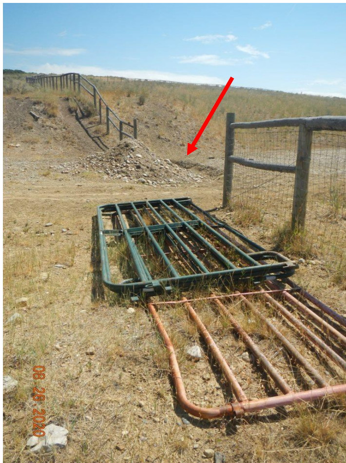
Photo#4: Gates down at entry. Arrow at point where cattle guard must have been installed before removal.
