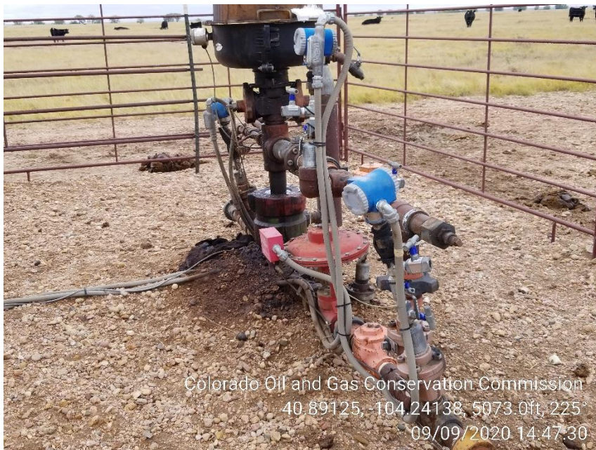
Photo 1 – Stained Soil at the Wellhead
