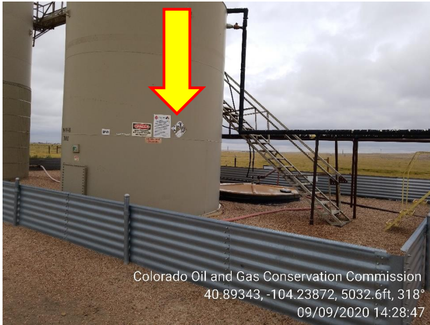
Photo 3 – 300 BBL Crude Oil Tank – NFPA Label has faded; no longer visible
