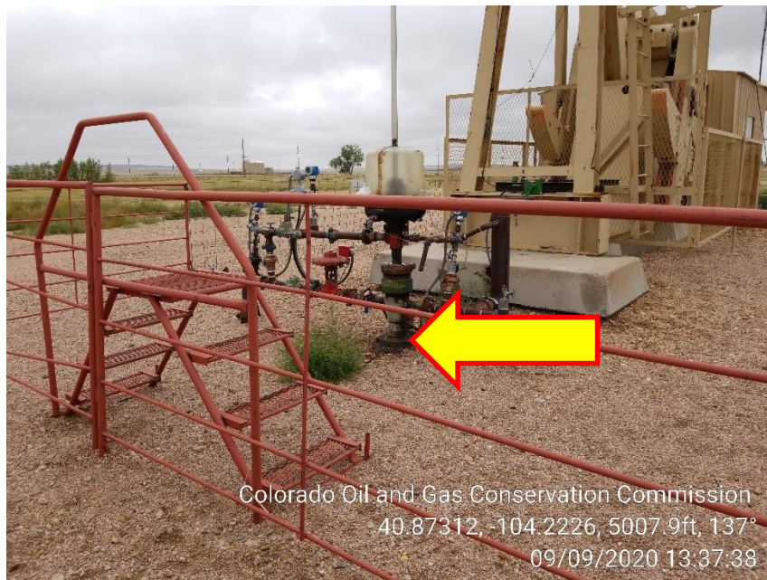
Photo 1 – Pumping Unit, Weeds, Stained Soil at Wellhead
