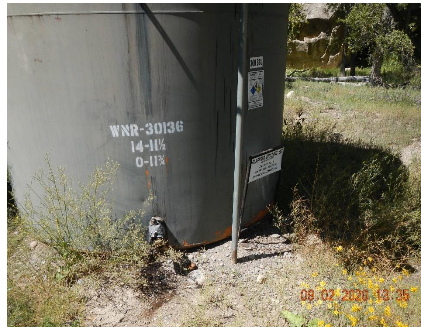
Stained soil beneath load out valve on north AST.
