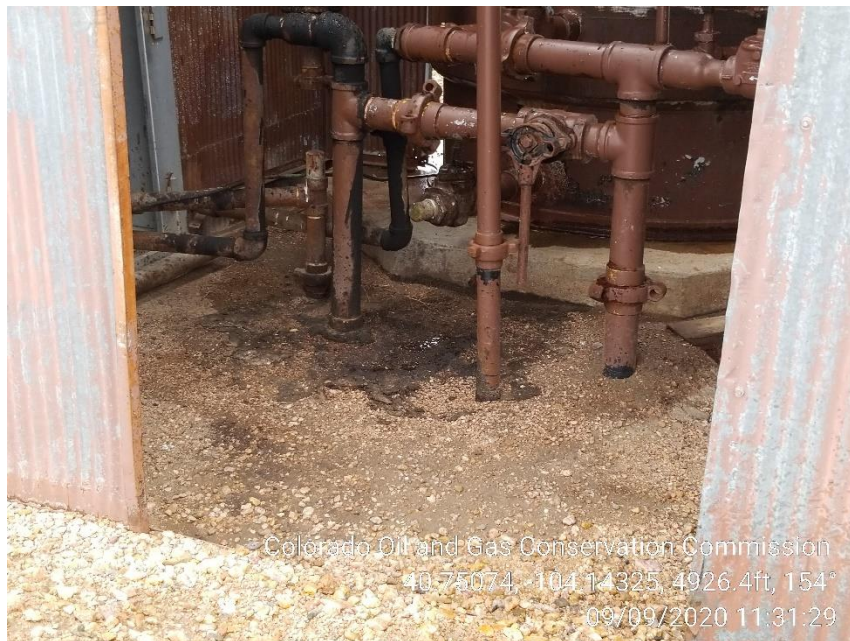
Photo 5 – Stained Soil at Heater Treater
