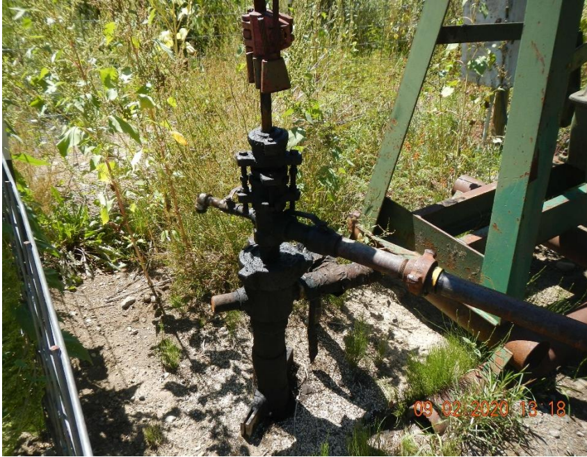
Well head is wet and stained.
