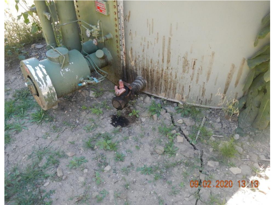
Stained soil beneath load out valve on eastern AST.
