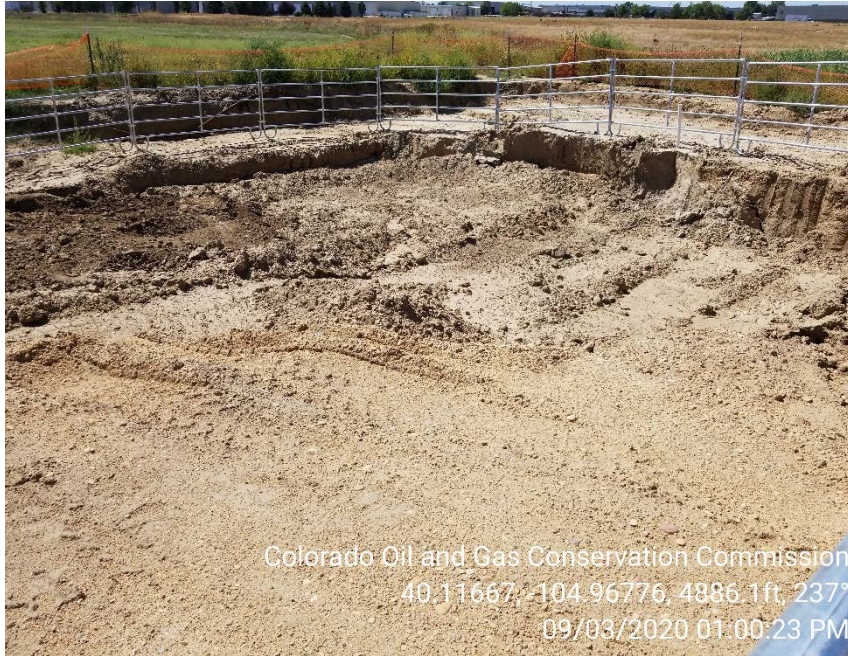
Photo 5 – Western excavation has been partially backfilled.
