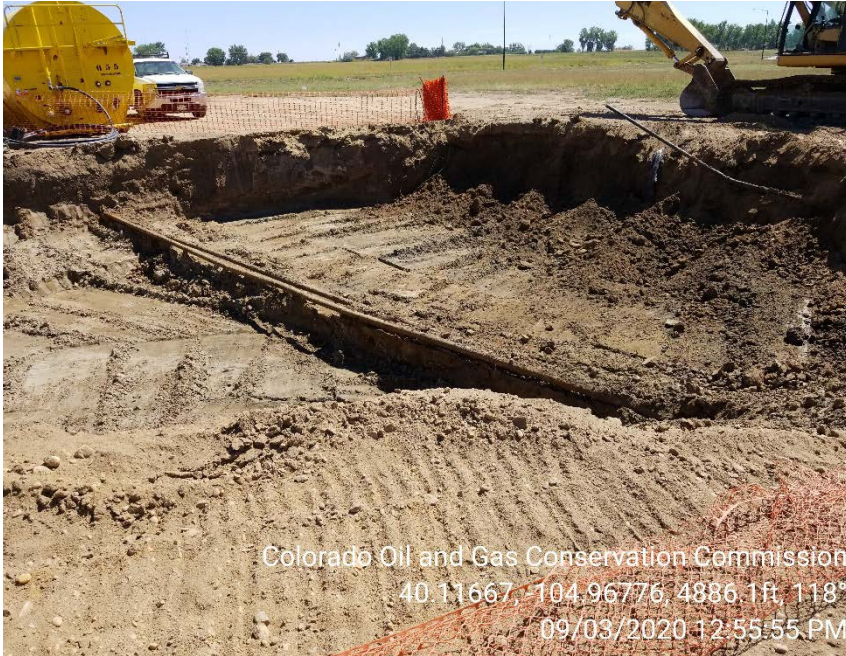
Photo 3 – Flowlines exposed in eastern excavation
