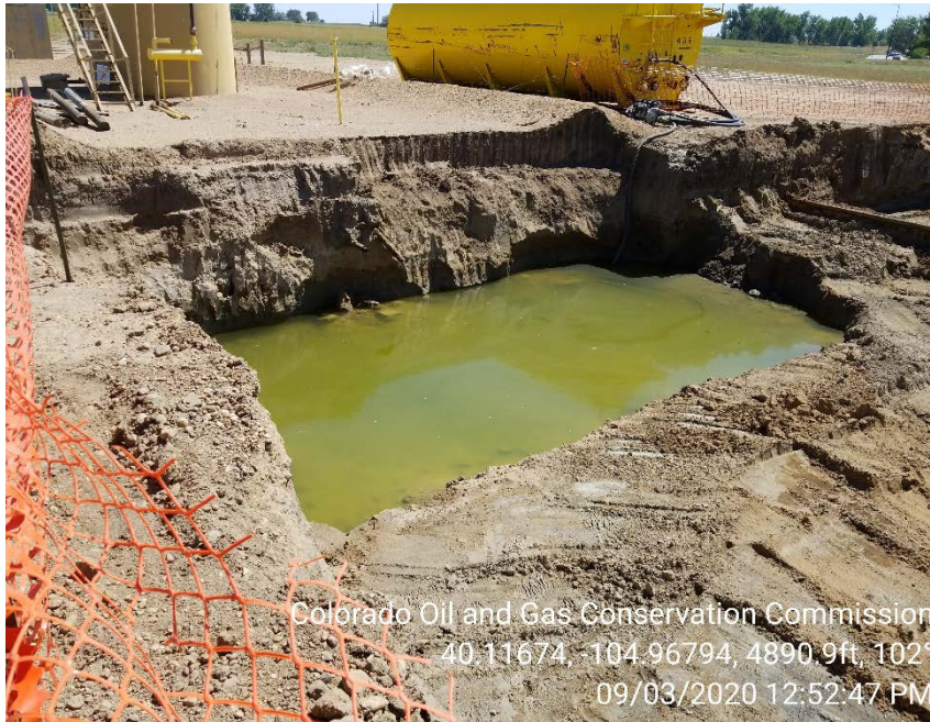
Photo 1 – Groundwater in northeast portion of the eastern excavation. Sheen observed on the water.
