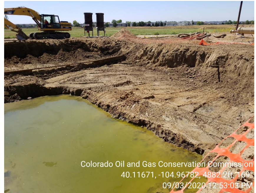
Photo 2 – South and west sidewall of eastern excavation. Flowlines exposed in portions of the excavation.
