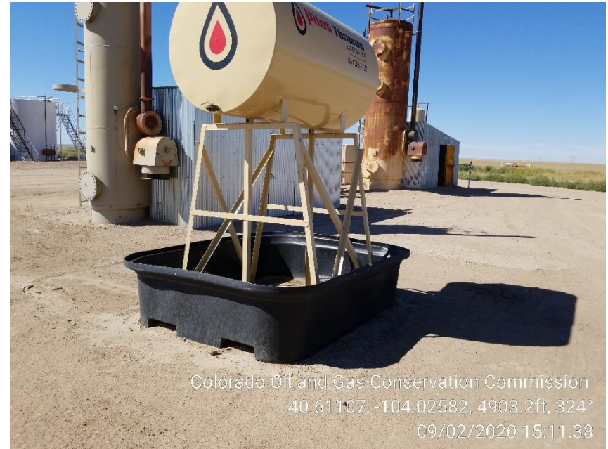
Photo 4 – Day Tank – missing Wildlife Netting
