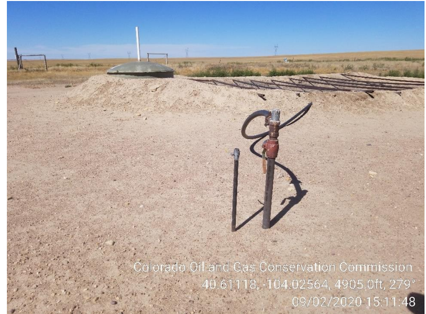
Photo 6 – Unmarked Riser South of Pit
