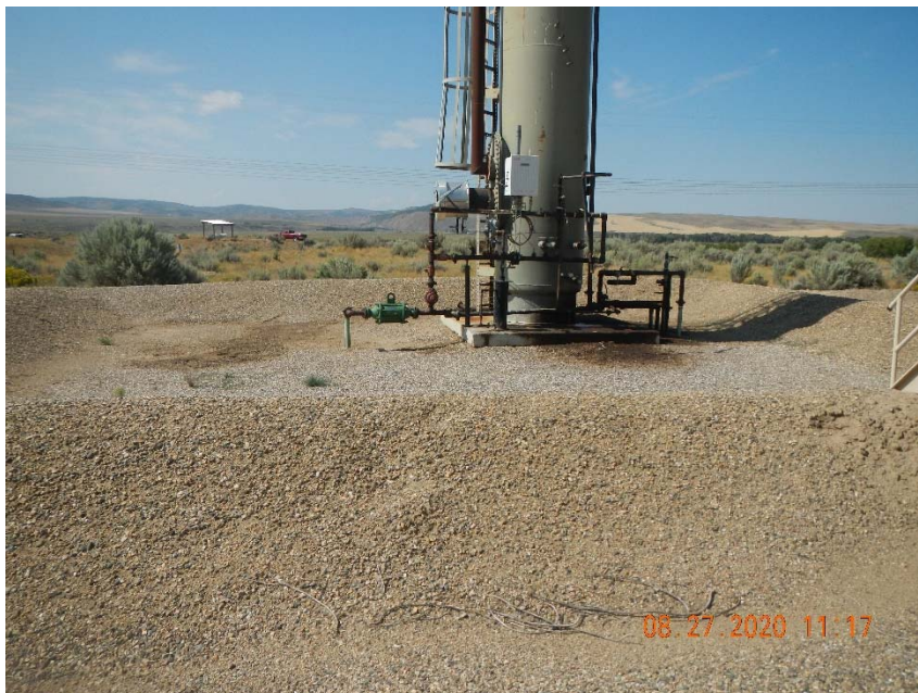
Photo 2. Stained soil at separator.
