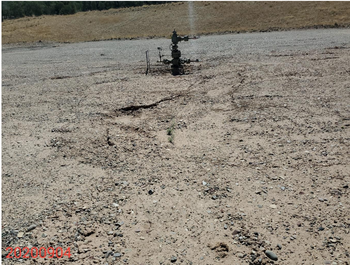
Photo 5: Photo taken from the north end of the Location, facing south. Photo show example of areas where subsidence concerns are evident on the Location.
