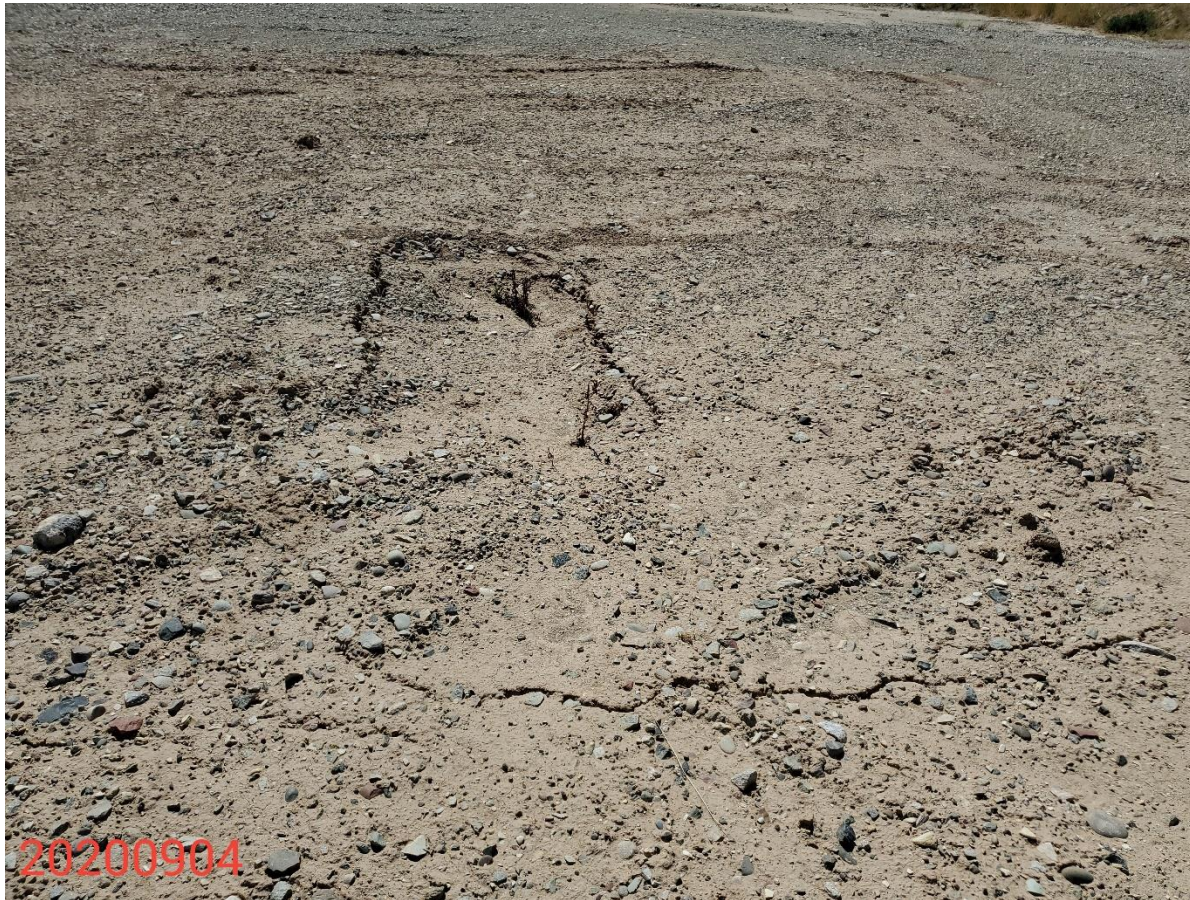
Photo 6: Photo taken from the west end of the Location, facing south. Photo show example of areas where subsidence concerns are evident on the Location.
