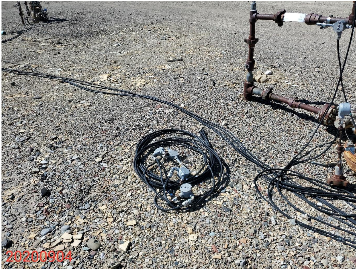
Photo 5: Photo shows what appears to be pressure gauges and tubing associated with the PA well. Equipment is unused and requires removal.
