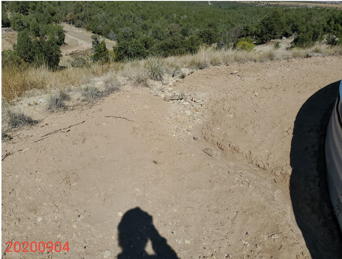
Photo 7: Photo taken from the northwest end of the Location, facing north. Photo shows erosion degradation due to stormwater runoff from the Location.
