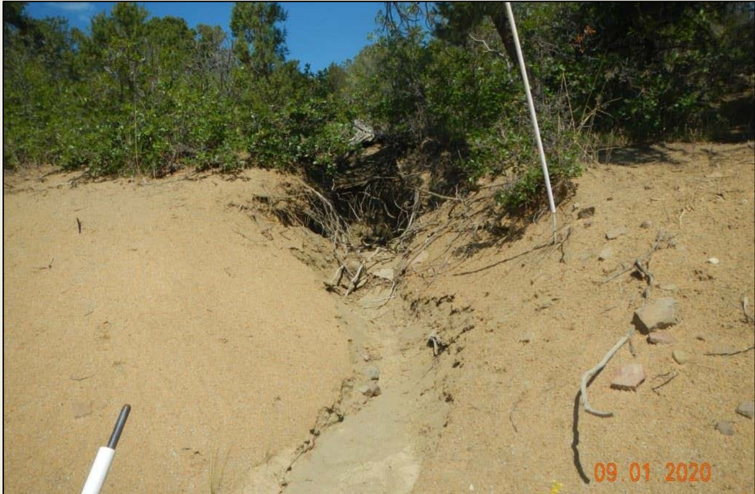
Photo 2. View of erosional channel approximately 3-5 feet wide and deep, within the northern cut-slope. Stabilization measures are needed here as significant erosion is observed.
