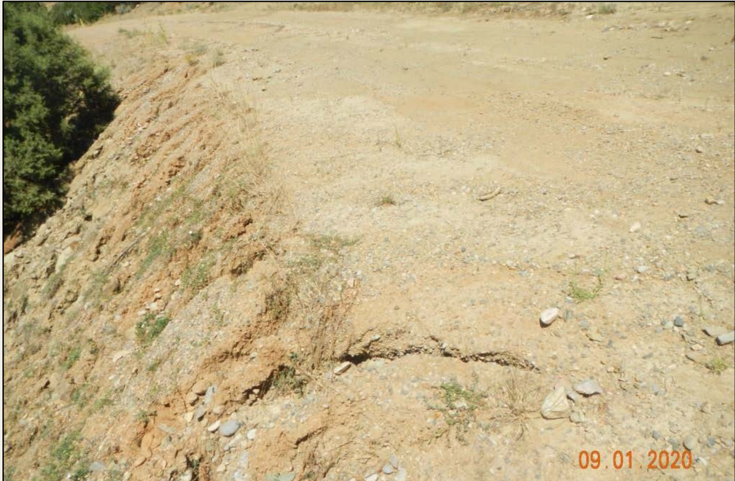
Photo 5. View of deep (~1 ft) rilling and scouring occurring along the access road where it appears that a recent storm event has recently caused significant erosion. BMPs along the access road need maintenance and repair,
