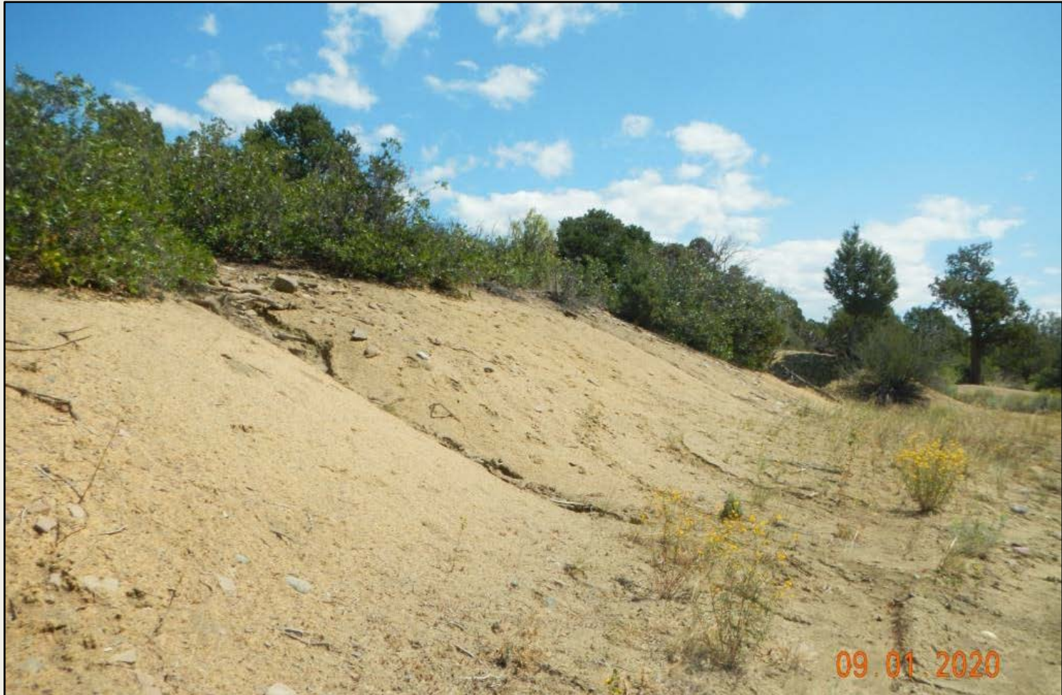
Photo 1. View of the northern cut-slope facing northeastward. Area is hydromulched, erosion and revegetation need to be monitored here.
