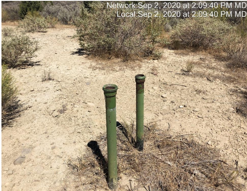
Photo #1839 flow line risers not LO/TO.
