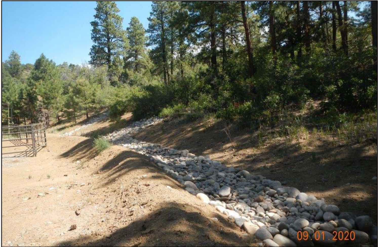
Photo 3. View of the eastern project area facing northward. Stormwater controls including cobble run-down, are installed.
