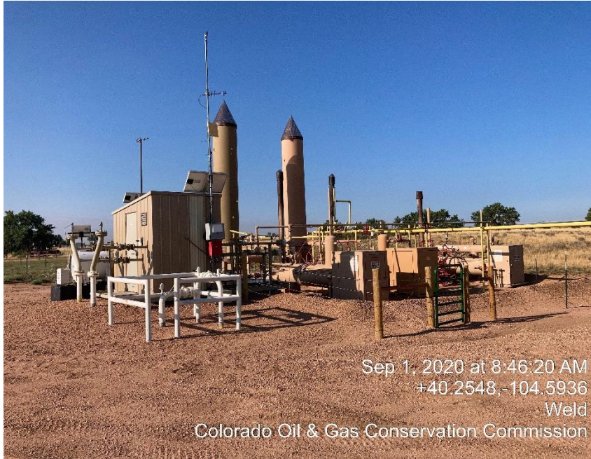
Photo #2 Separators, ECD's & Meter Runs
