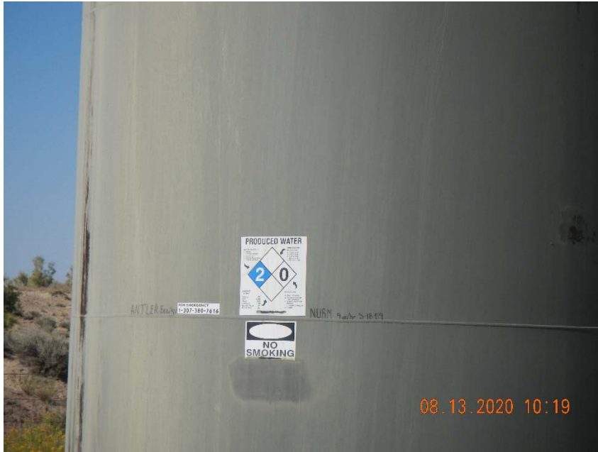
Photo 2. Example of incomplete and faded tank label.
