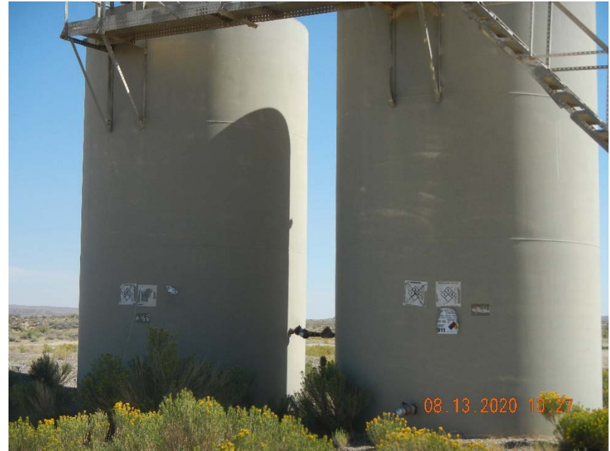
Photo 3. Example of faded, incomplete, peeling tank labels.
