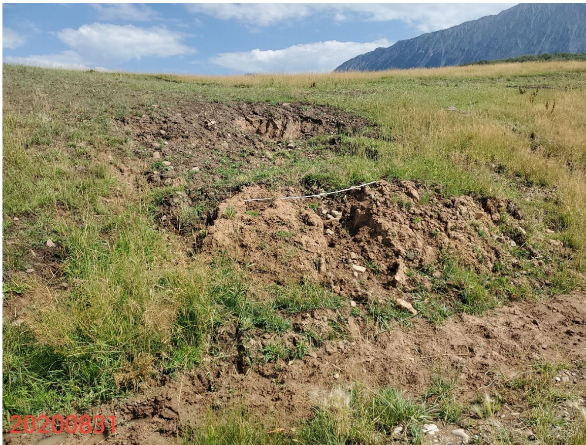
Photo 13: Photo taken from the cut slopes on the north end of the Location. Photo shows Operator has failed to implement BMPs to protect and stabilize slopes; erosion degradation has continued. 6 foot measuring stick for reference.
