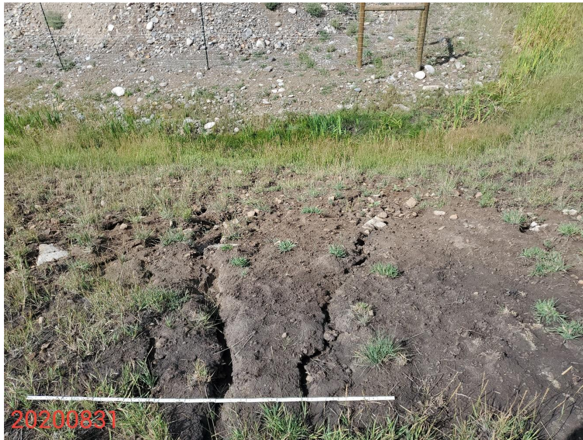
Photo 16: Photo taken from the cut slopes on the northeast corner of the Location. Photo shows BMPs remain missing or insufficient to stabilize and protect slopes. 6 foot measuring stick for reference.
