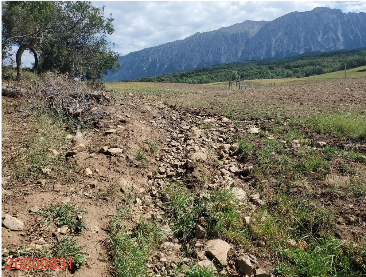
Photo 8: Photo taken from the ditch on the northwest end of the Location, facing east. Photo shows stormwater erosion has continued and appears to have removed the soils and finer particulates on areas of the Location and the ditch.
