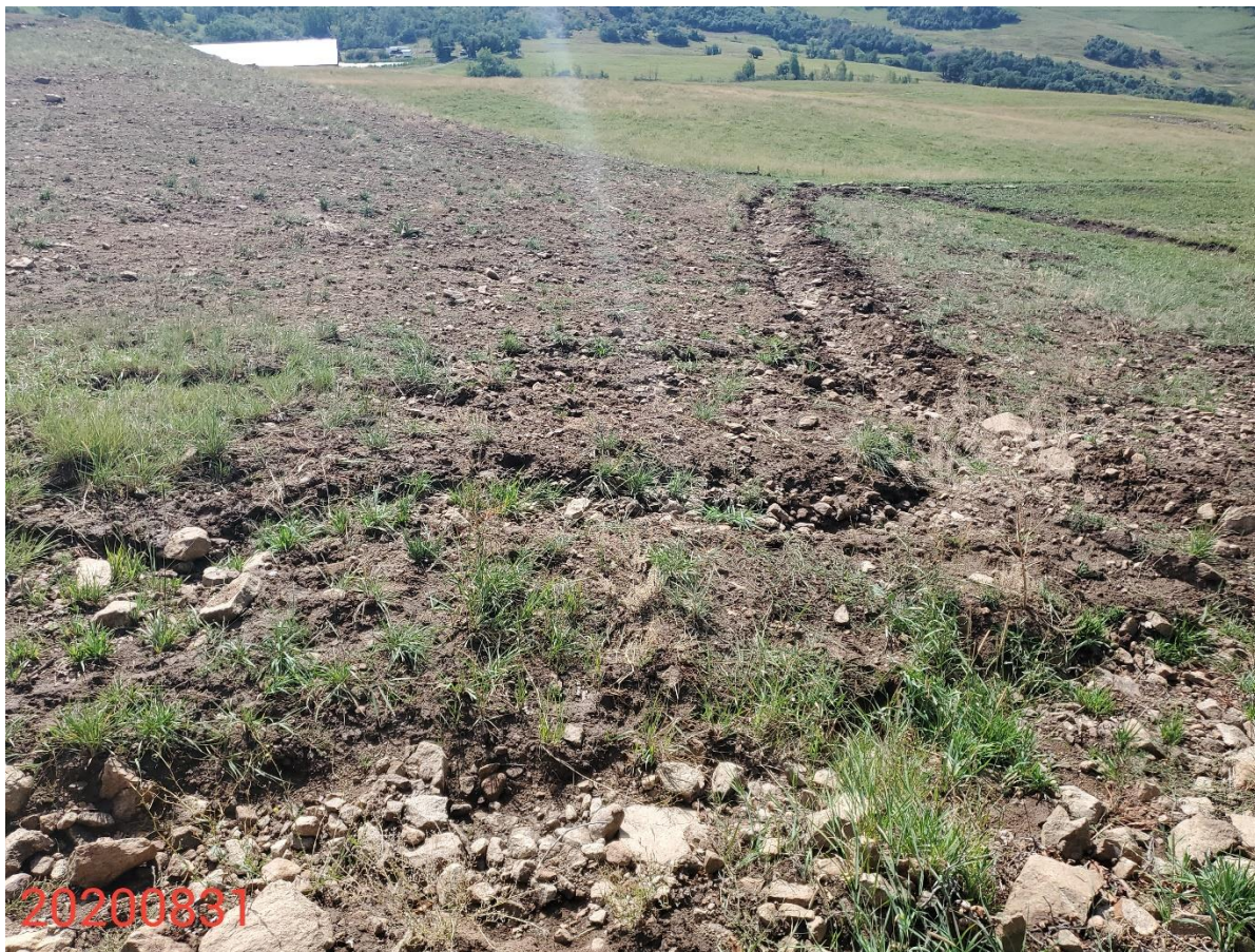
Photo 7: Photo taken from the northwest end of the Location, facing south. Photos shows ditch BMP. BMPs appears insufficient, as stormwater degradation due to runoff is evident below BMPs evident
