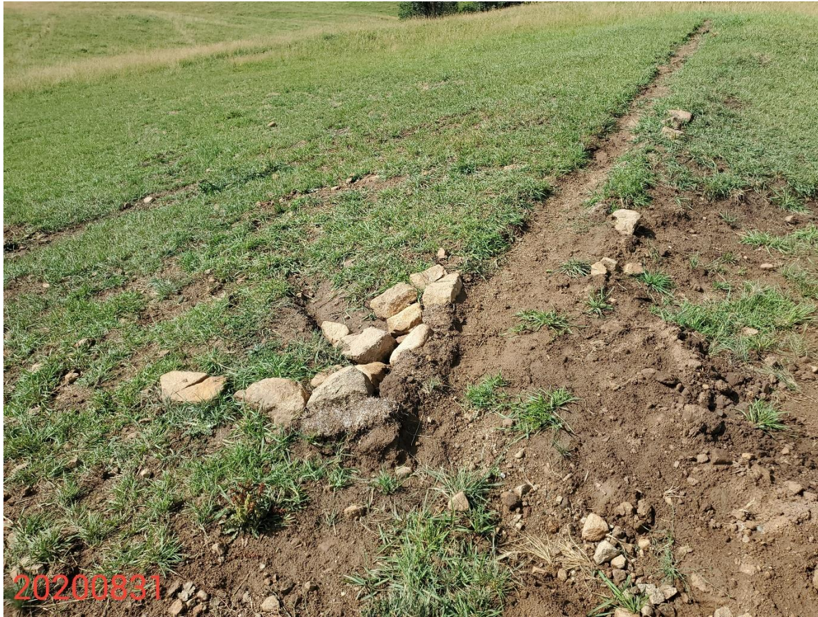
Photo 6: Photo taken from the Ditch BMP on the west end of the Location. Photo shows Operator appears to have installed a velocity check as an outlet; This does not appear to be a sufficient or appropriate long term outlet to allow for sediment laden-free stormwater discharge.
