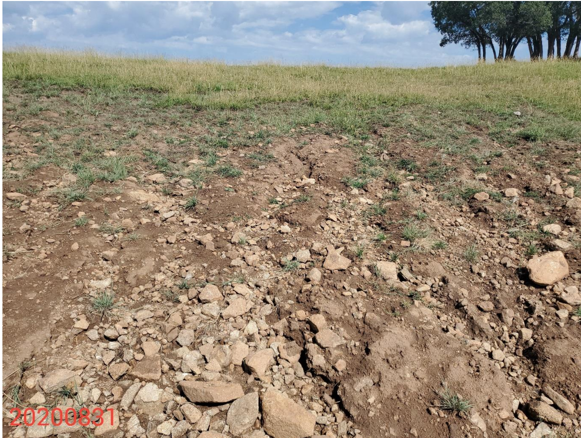
Photo 9: Photo taken from the northwest end of the Location, facing north. Photo shows where topsoil was stored. Photo shows BMPs remain missing, or insufficient to protect slopes, and erosion degradation has continued resulting in loss of soils.
