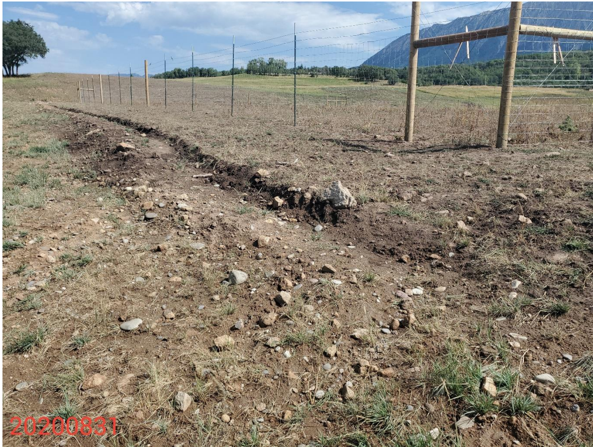
Photo 3: Photo taken from the southwest corner of the Location. Photo shows perimeter stormwater ditch. Ditch BMP has not been constructed in accordance with good engineering practices; BMP ends on the southwest end of the location and does not have a sufficient outlet to allow for sediment laden-free stormwater discharge.
