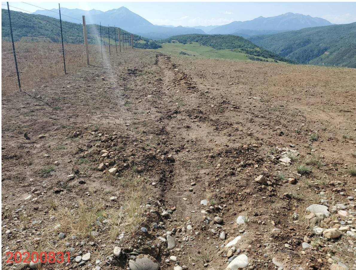
Photo 12: Photo taken from the northwest corner of the pad, facing south. Photo shows stormwater ditch is filling with sediment.
