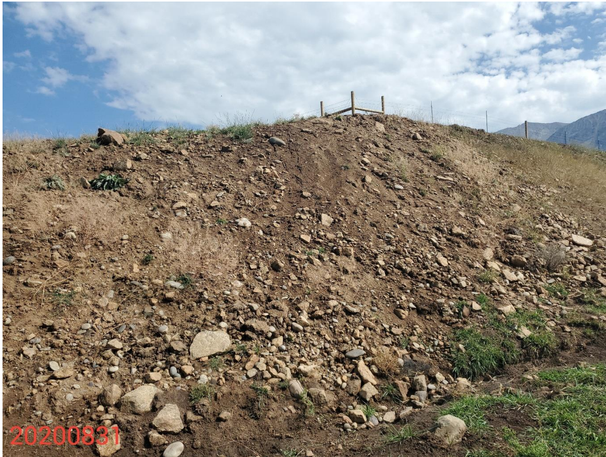
Photo 4: Photo taken from the from the southwest end of the Location, below ditch in photo 3. Photo shows Operator appears to have repaired the erosion degradation documented in the 5/26/2020 inspection. However, BMPs remain insufficient or missing to protect the slopes, and to allow for sediment laden-free stormwater discharge from the ditch
