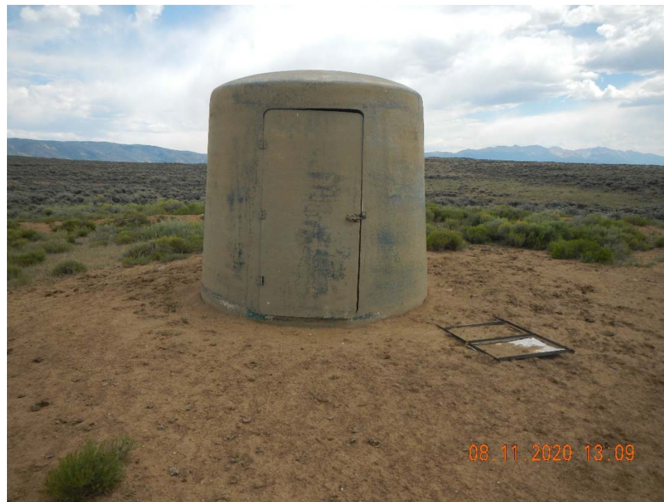
Photo 1. Wellhead sign knocked over. Door to housing stuck shut.
