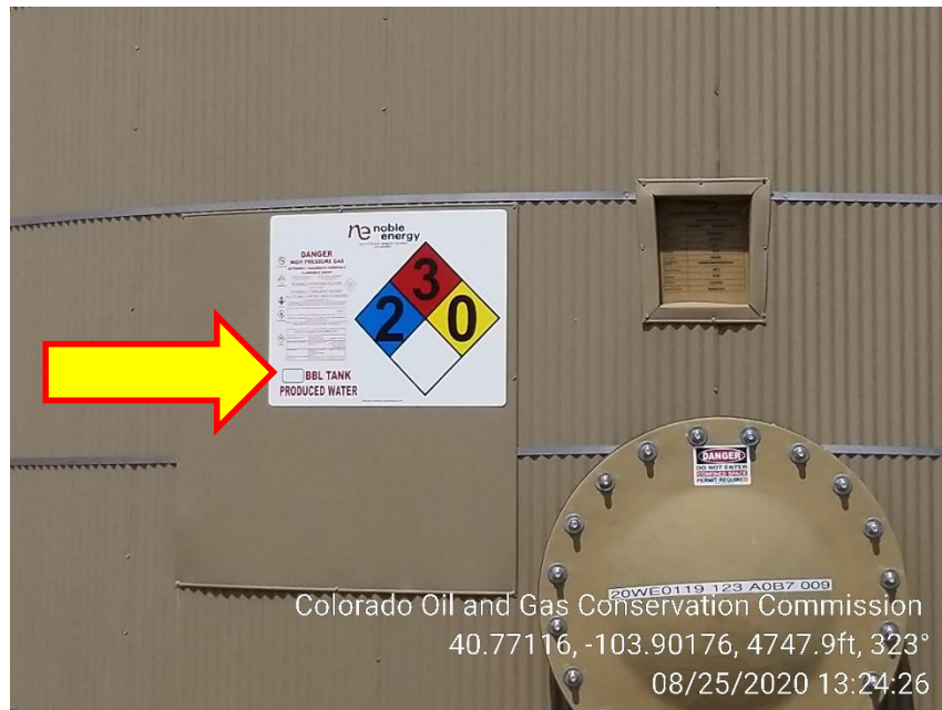
Photo 7 – Produced Water Tanks, Missing Capacity
