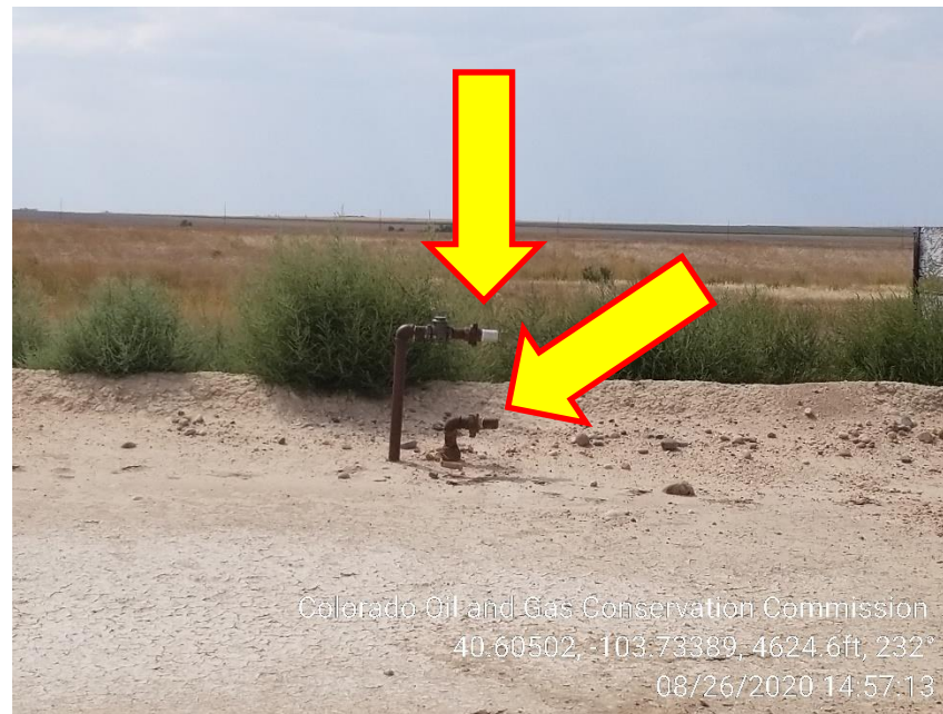
Photo 10 – Unmarked Risers at Tank. Weeds
