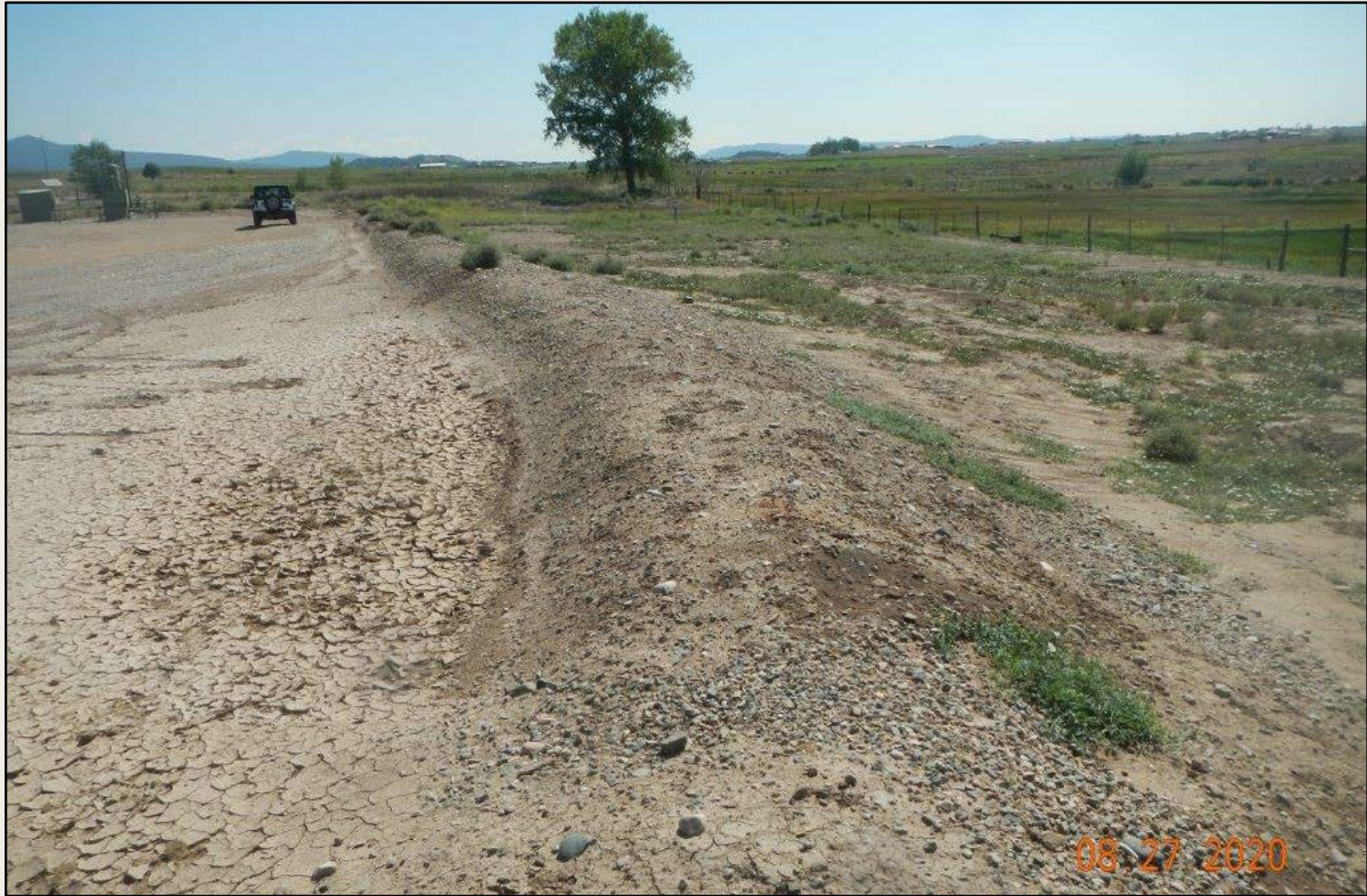
Photo 2. View of the southern fill slope. Berms are installed. Erosion channels are graded and appear to be seeded.
