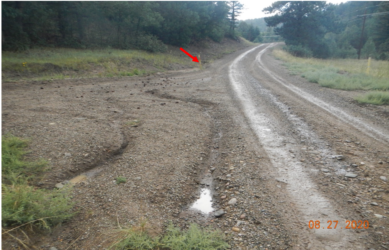
Photo 2. There is a plugged culvert along the main road (red arrow) causing stormwater to flow down the road. Lat/Long:37.09178,-104.93688.
