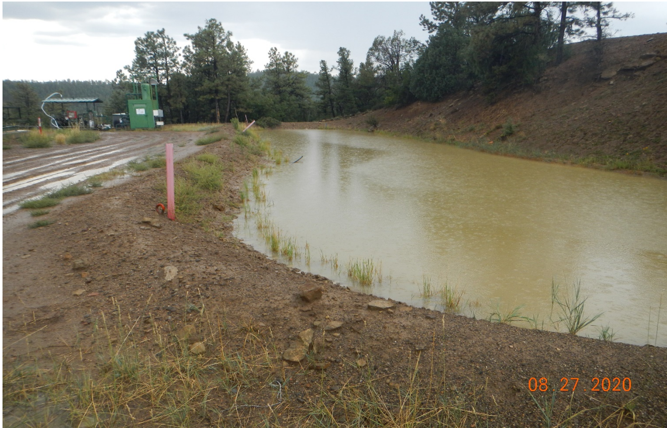
Photo 8. The water in the pit is approaching 2 ft. freeboard.
