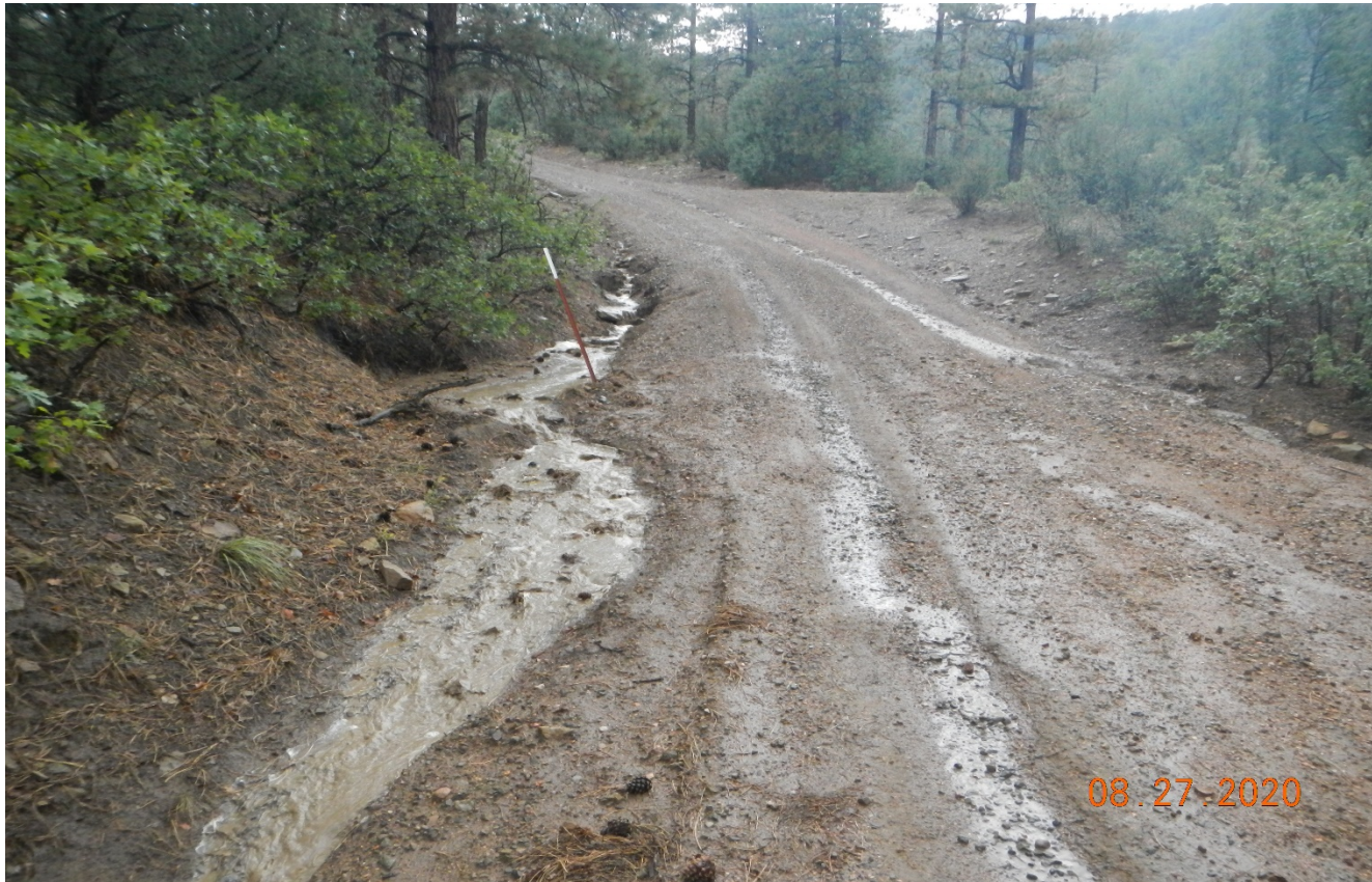
Photo 6. The culvert is plugged up along the road causing stormwater to flow down the road as shown in the previous photo.
