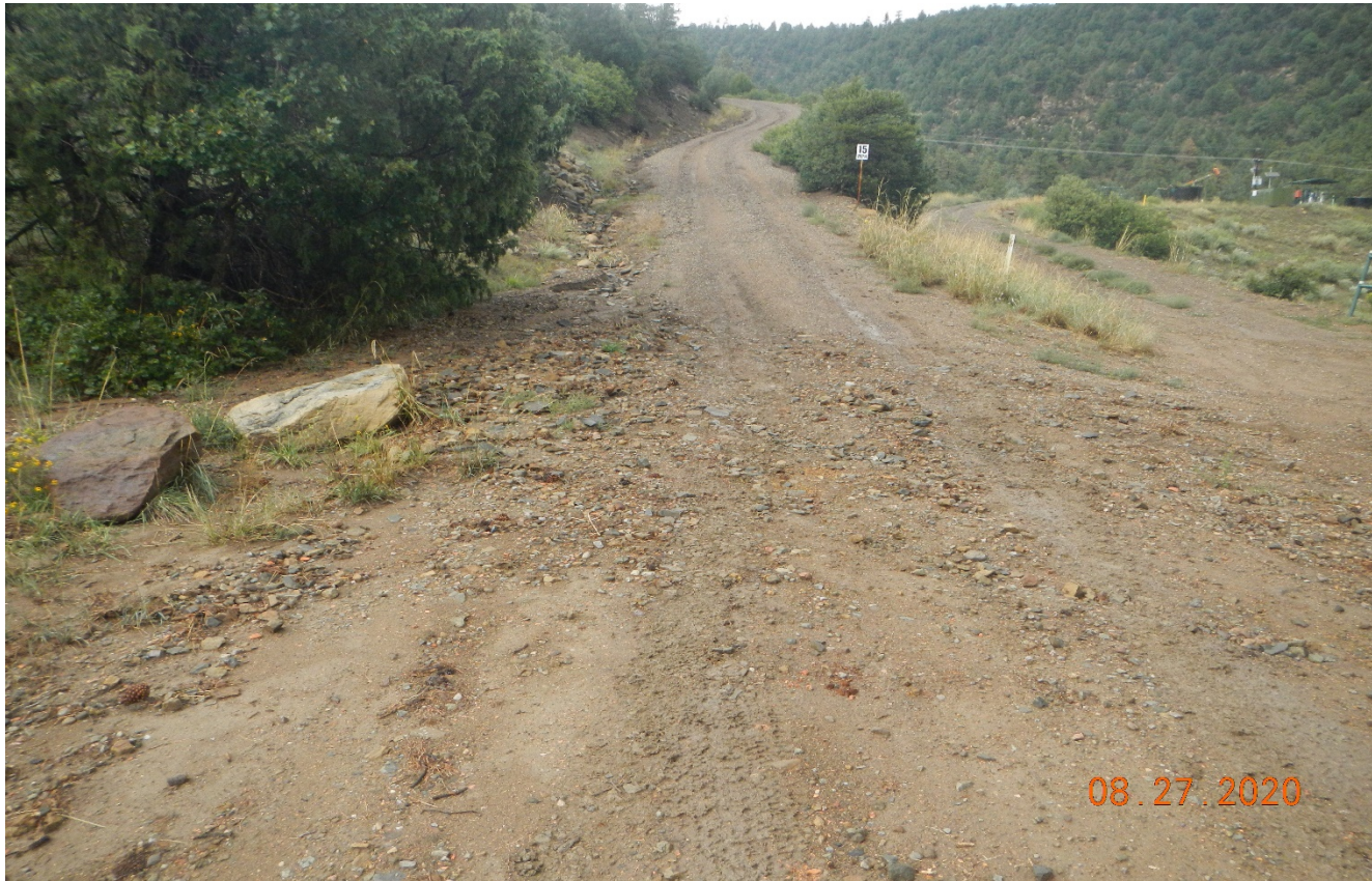
Photo 3. There is sediment accumulation at the bottom of the road which appears to be coming uphill from the access road or pipeline area.
