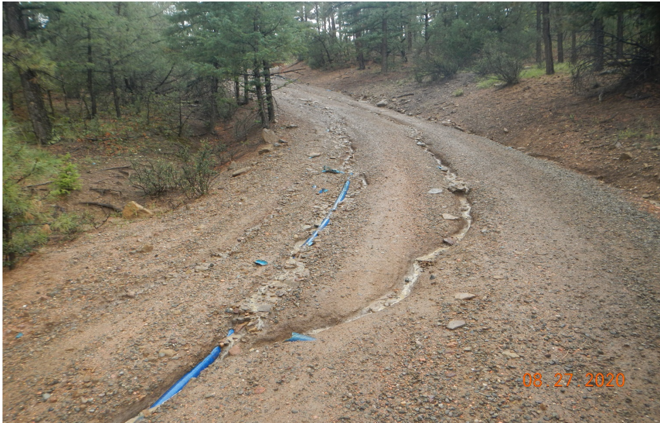
Photo 7. Facing southwest along the access road. There is erosion occurring down the road. The blue plastic debris from pipe should be picked up.
