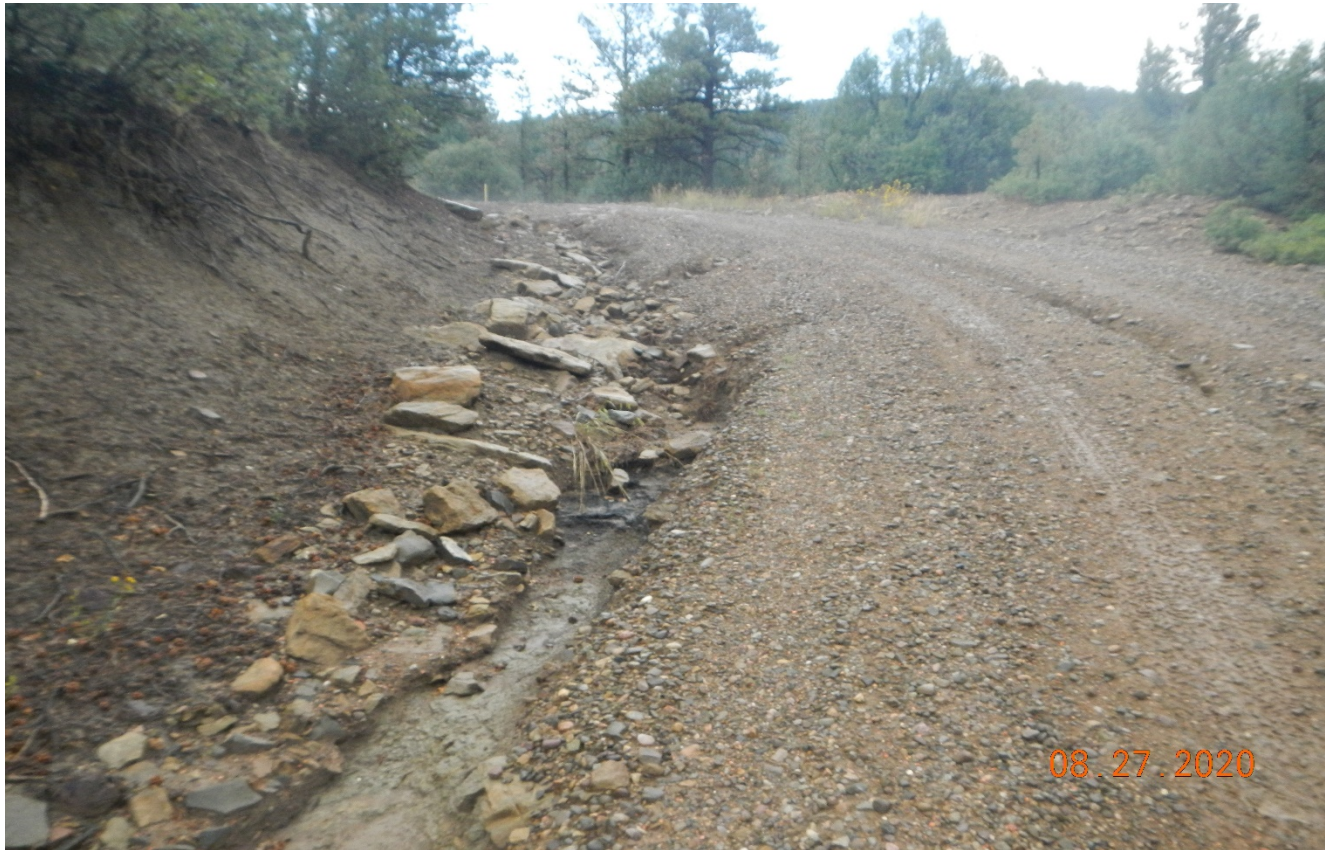
Photo 4. BMP's are needed along the side of the road to dissipate stormwater flow.
