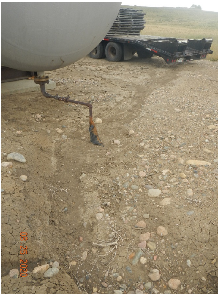
Photo#6: Sediment migration & developing erosion at West side of Location.
