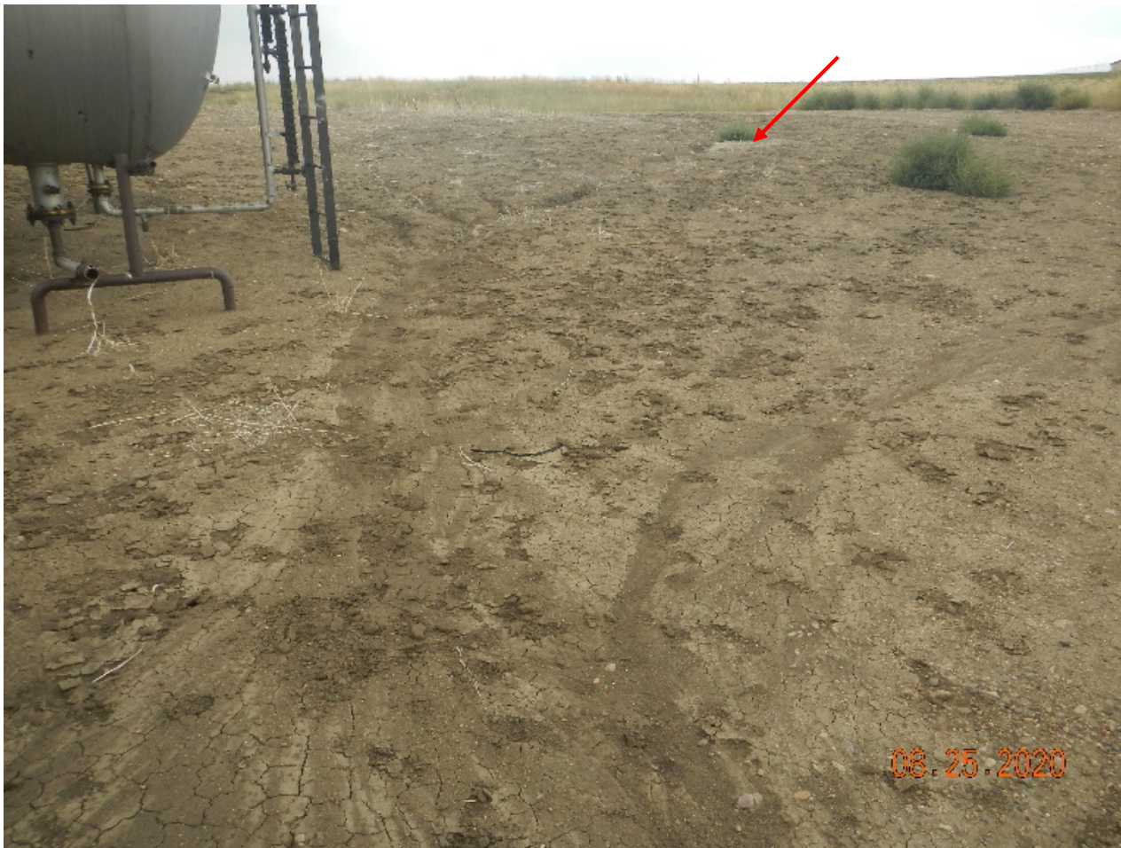
Photo#8: Sediment migration & developing erosion at West side of Location.
