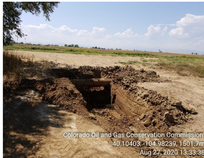
Photo 2 Crew onsite exposing a gas leak just to the west of well head.
