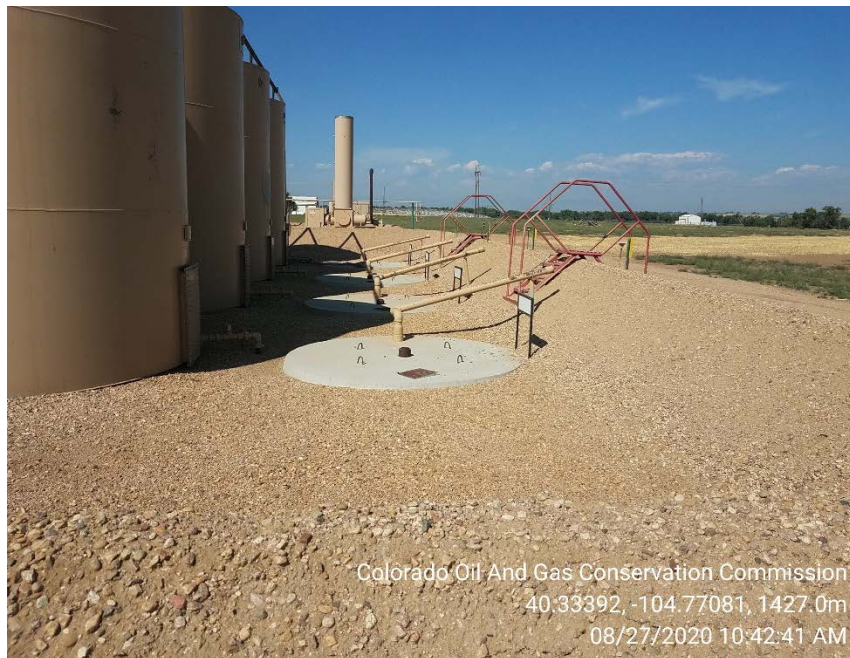
Unused produced water vaults
