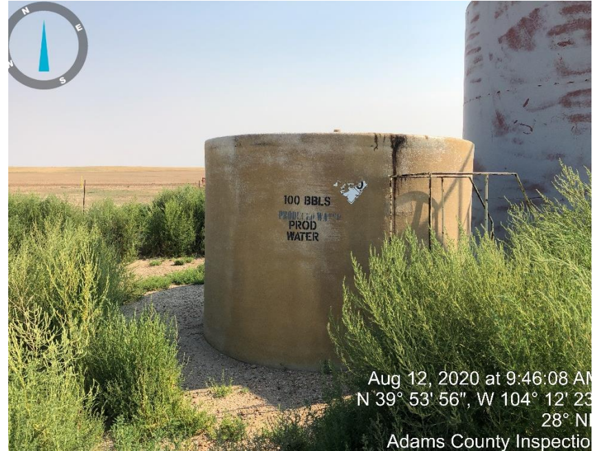
Photo #2 Produced water tank.
