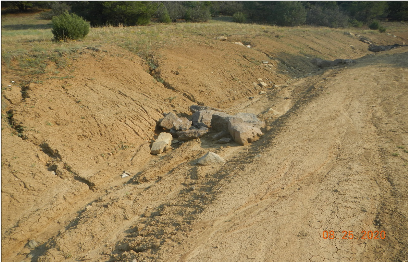
Photo 2. There are rocks piled up for a check dam however, this is not an adequate installation of a check dam. There is erosion along the side slopes of the road which needs to be seeded and stabilized.
