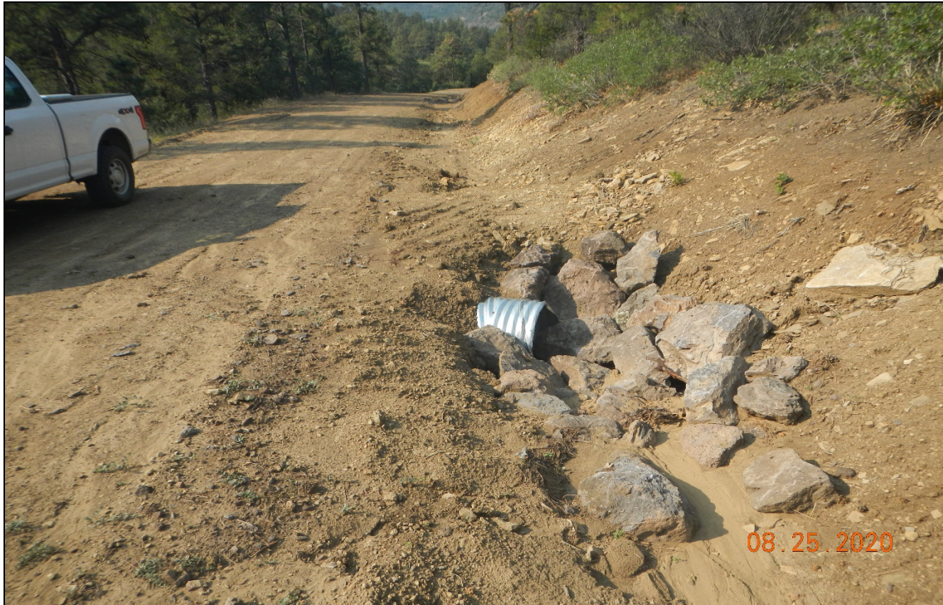
Photo 8. This is a view of another culvert further along the road which the rock is obstructing the culvert inlet.
