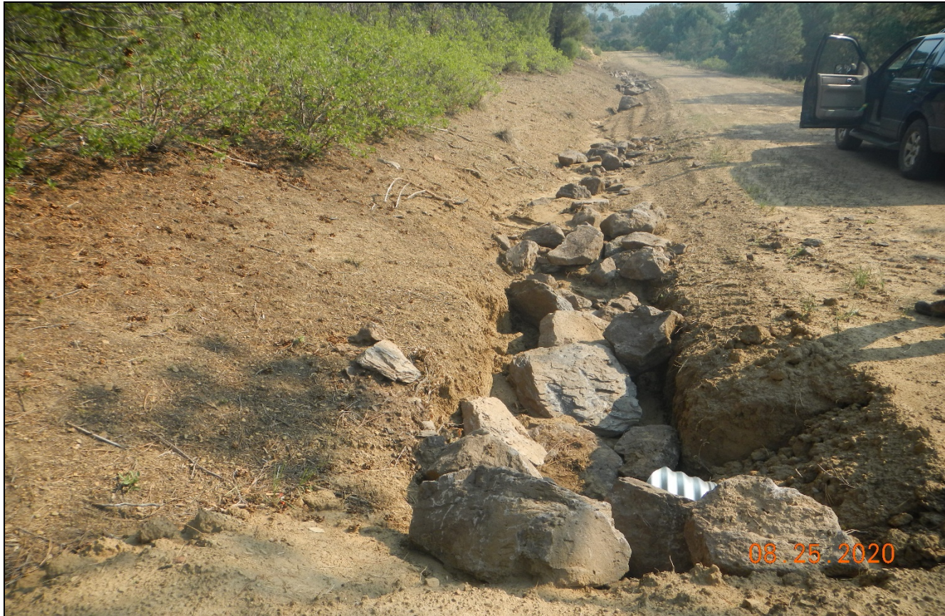
Photo 10. There is large rock rip/rap installed in front of the culverts which may obstruct the culvert inlet.
