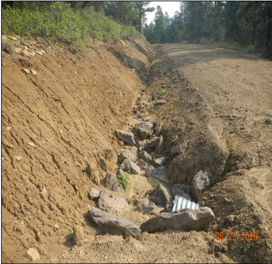
Photo 6. Additional culverts were installed along the road but rock rip/rap is piled in front of the culverts which could block up culvert inlets.
