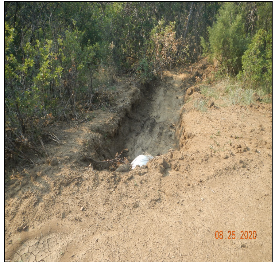
Photo 4. There is no outlet protection installed at the culverts which could cause erosion.
