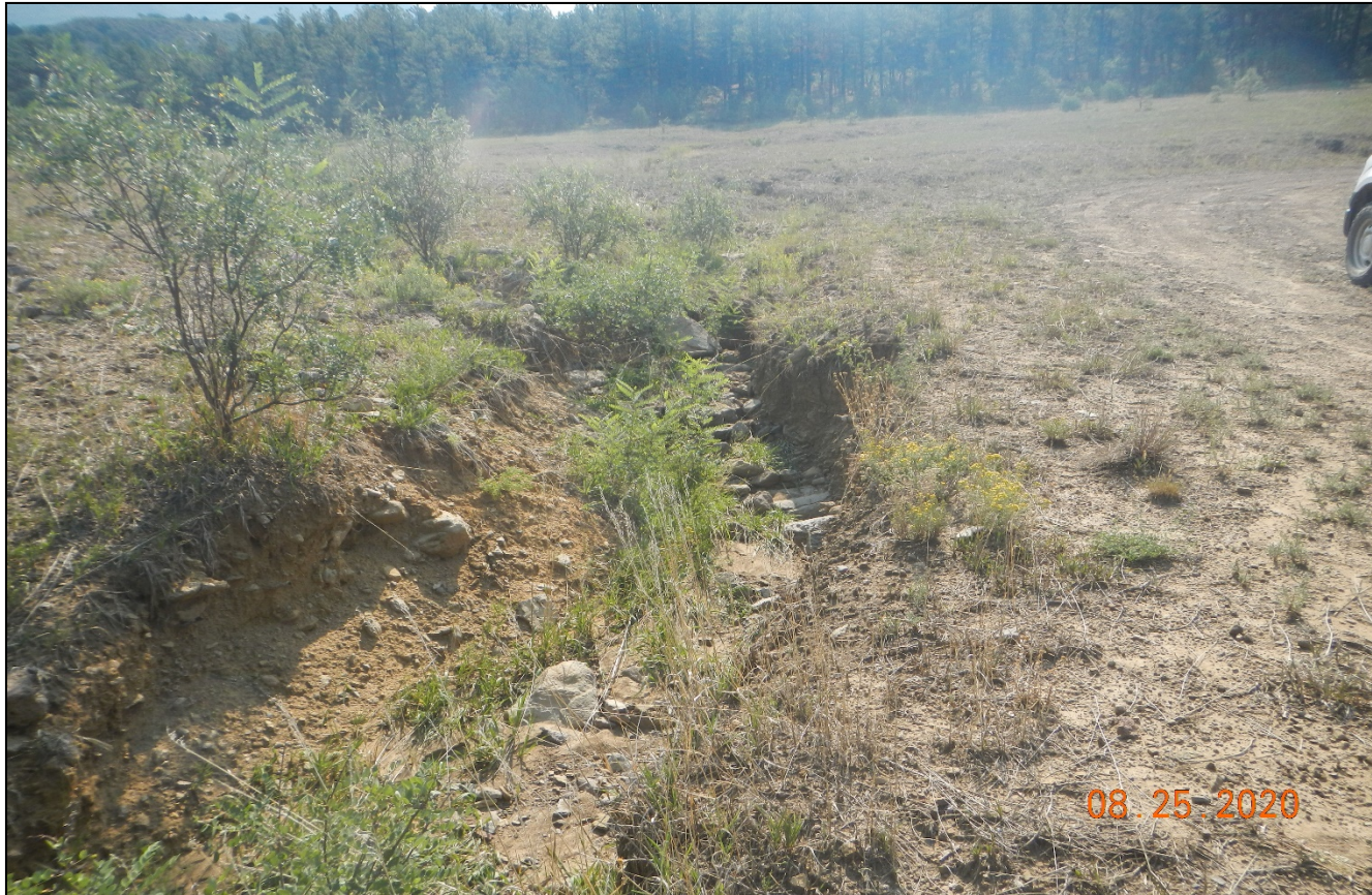
Photo 19. There is an erosional gully along the access road that was not repaired at Lat/Long:37.02219,-104.48216.
