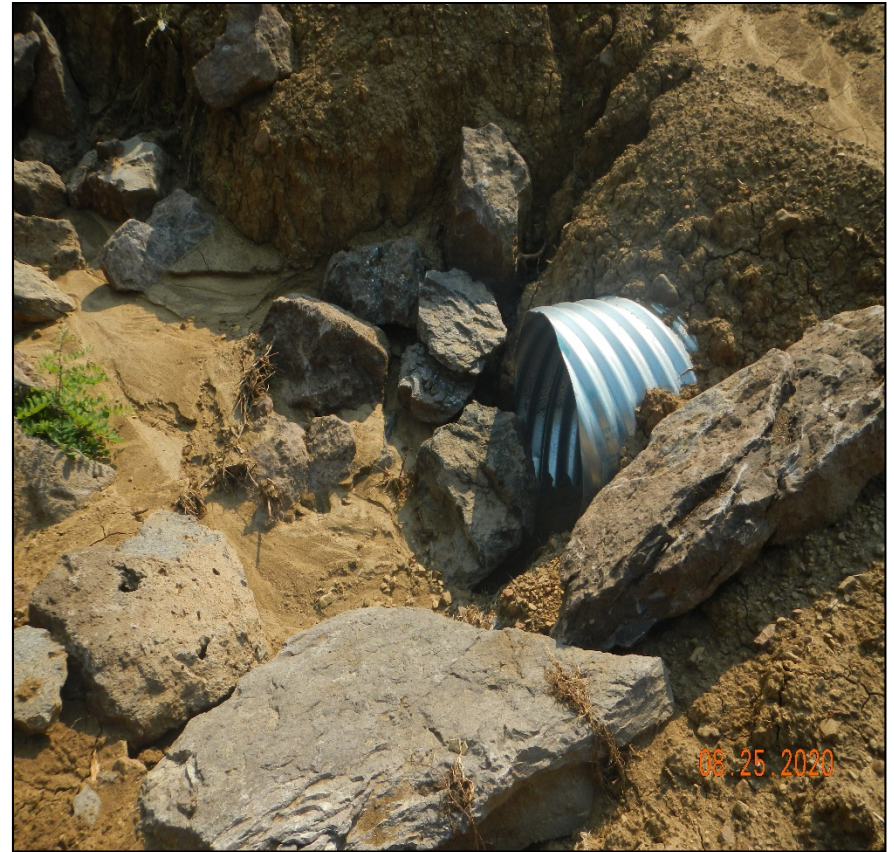
Photo 7. This photo shows the rock obstructing the culvert inlet.
