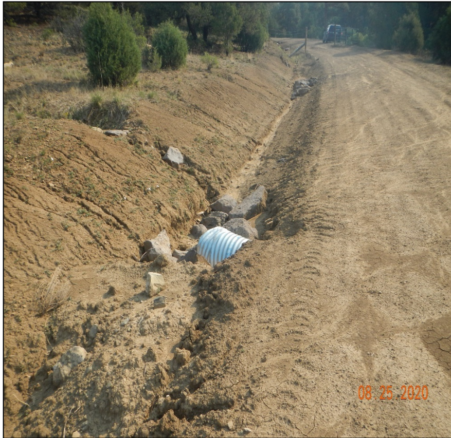
Photo 3. Additional culverts were installed along the road but rock rip/rap is piled in front of the culverts which could block up culvert inlets.
