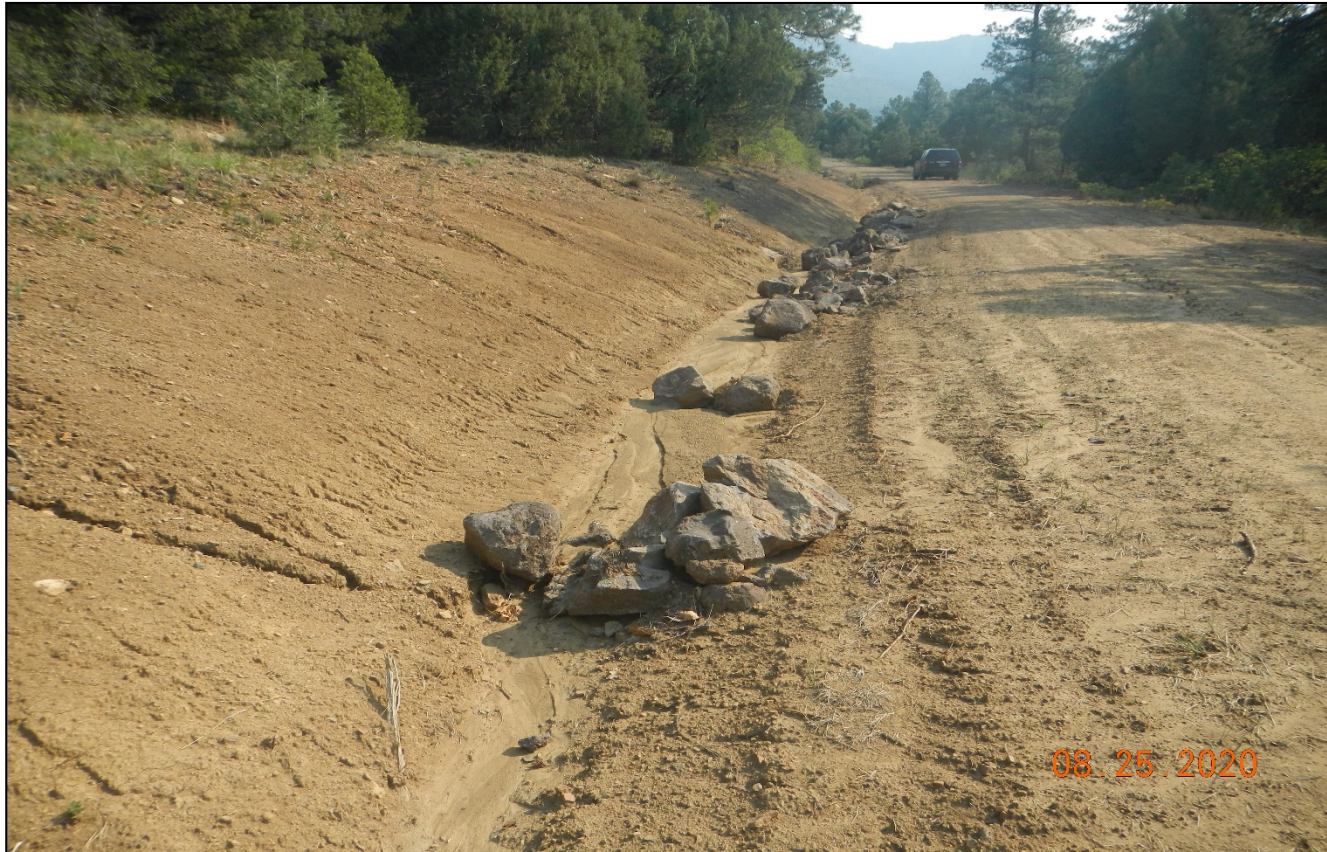
Photo 9. The rock was scattered along the side of the road and not properly installed. The side of the road will need to be seeded and stabilized.
