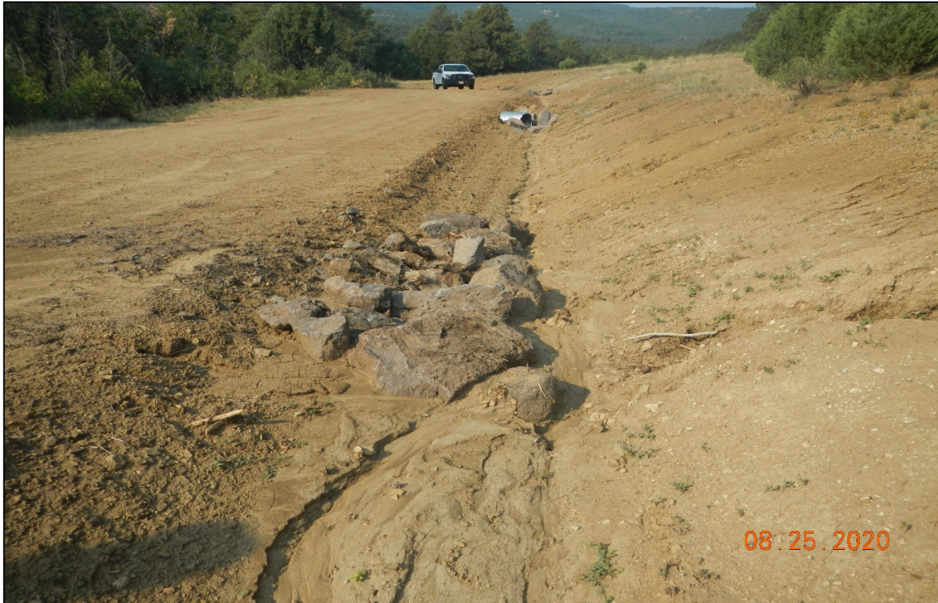
Photo 5. The rock check dam is not properly installed and there is signs that stormwater is flowing around the rip/rap. The check dams need to extend from side to side with the low point at the center of the check dam.
