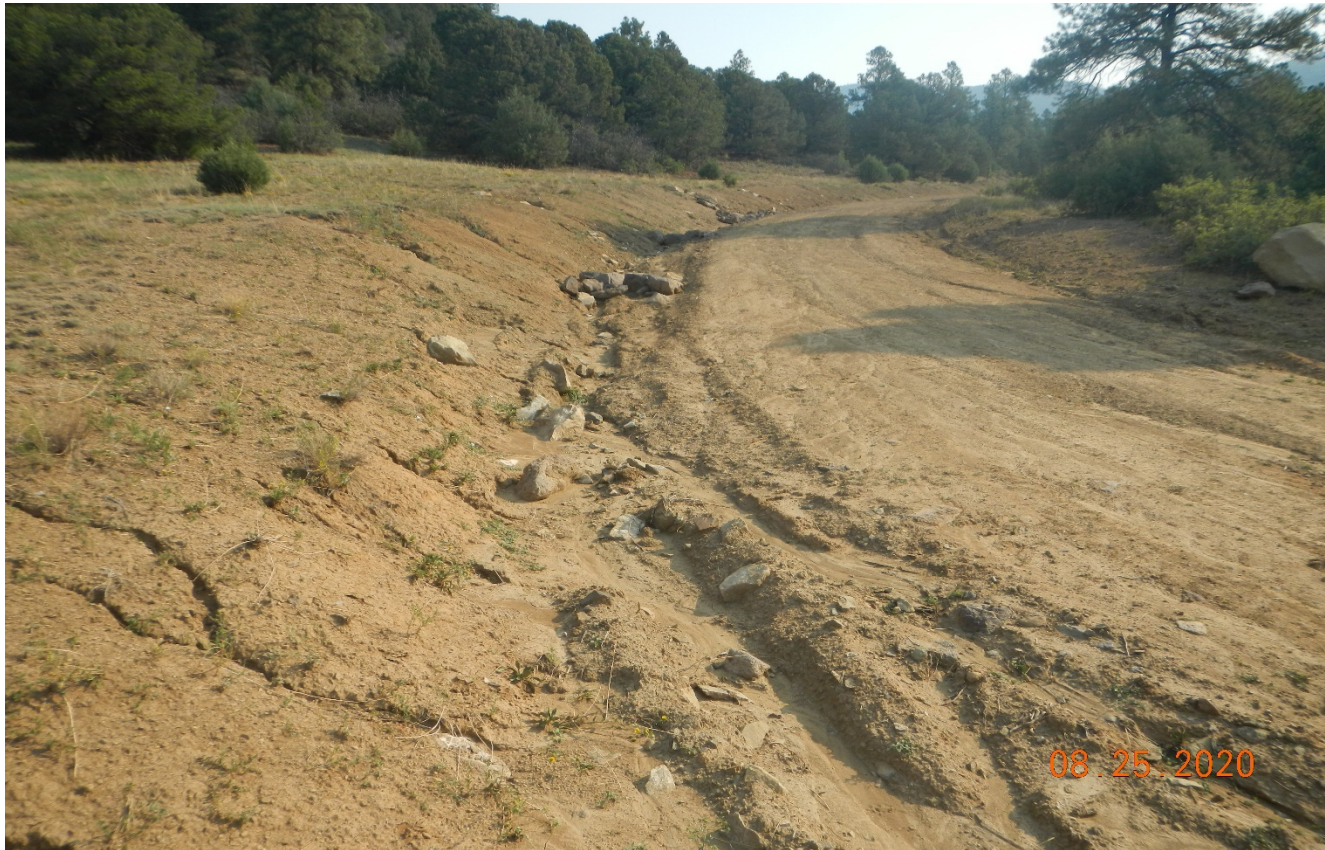
Photo 1. Facing northeast along the access road. The road has been regraded however, BMP's are not adequately installed and there are signs of erosion. The side slopes of the road will need to be seeded and stabilized.
