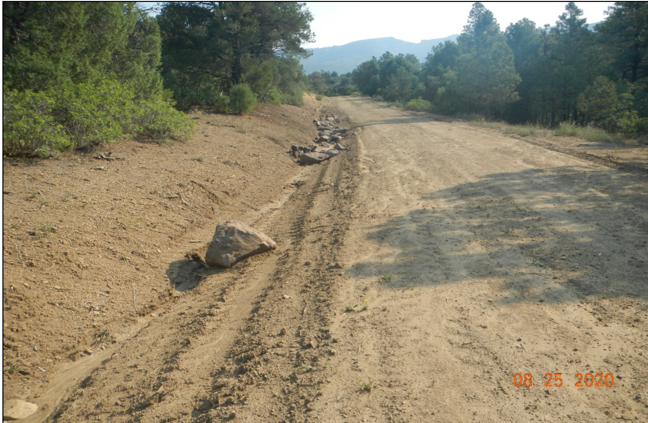
Photo 11. The rock was scattered along the side of the road and not properly installed. The side of the road will need to be seeded and stabilized.
