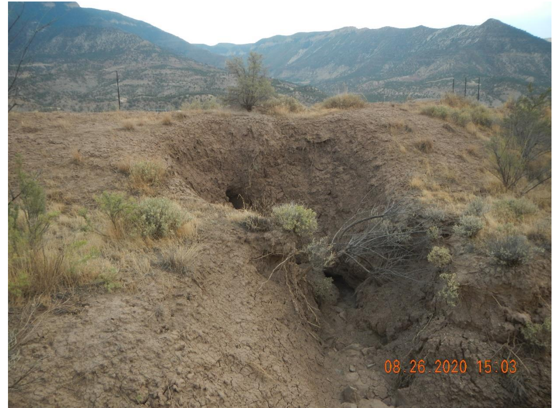
Channel thru berm behind separators.
