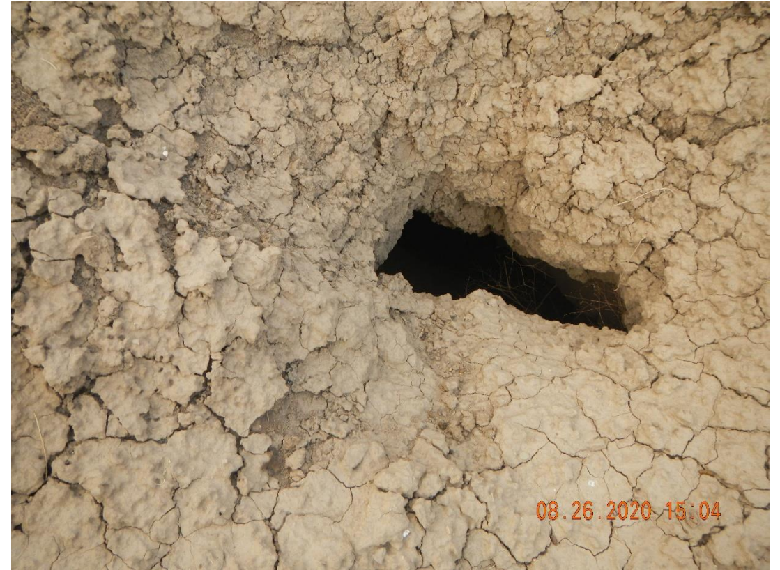
Channel thru berm behind separators.
