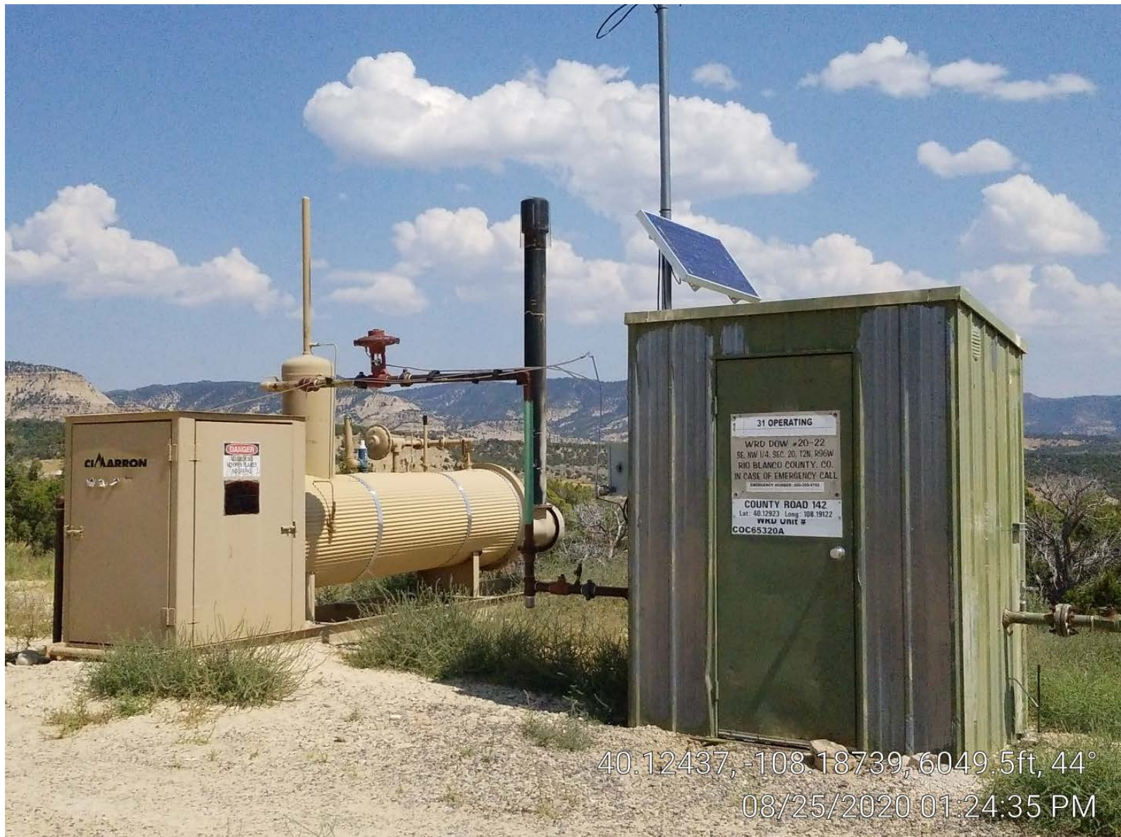
Photo 3. Separator & meter building.
