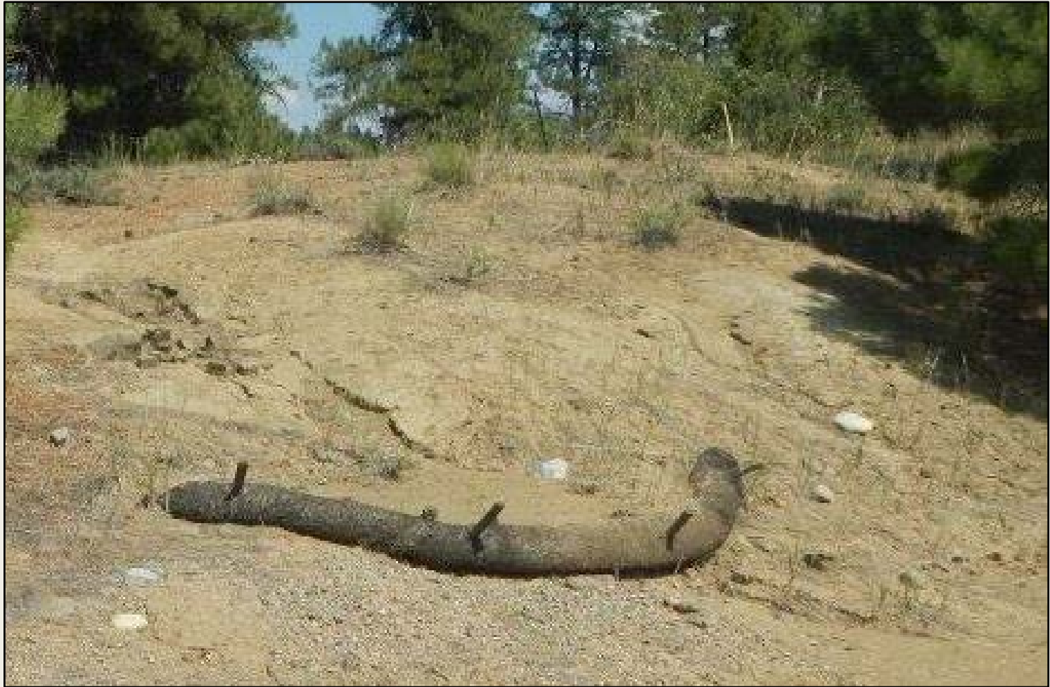
Photo 4. View of wattle on the northwestern cut-slope that is filled with sediment. Wattle does not appear to be an adequate BMP to stabilize this area.
