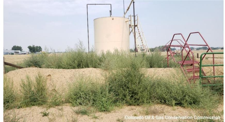
**Photo 3 weeds overgrown in tank berm**
