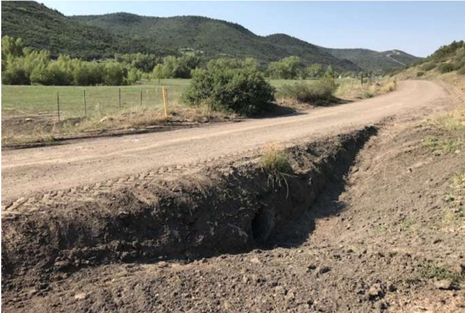
PHOTO 8: THE SEDIMENT ACCUMULATION WAS REMOVED FROM THE CULVERT INLET.
