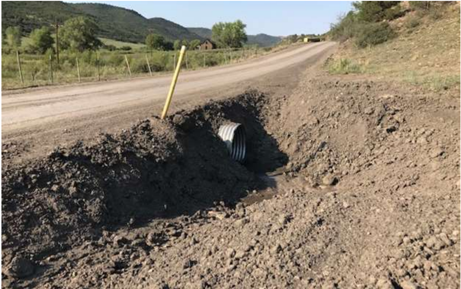
PHOTO 2: A NEW 36 INCH CULVERT WAS INSTALLED ALONG THE SOUTH FORK LEASE ROAD.
