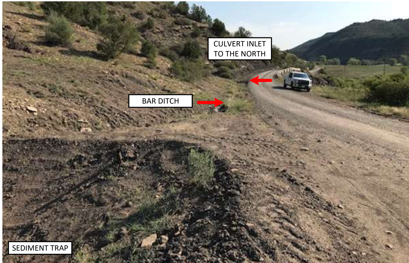
PHOTO 4: OVERFLOW FROM THE SEDIMENT TRAP IS DIRECTED TO THE CULVERT INLET DOWN GRADIENT OF THE SEDIMENT TRAP.
