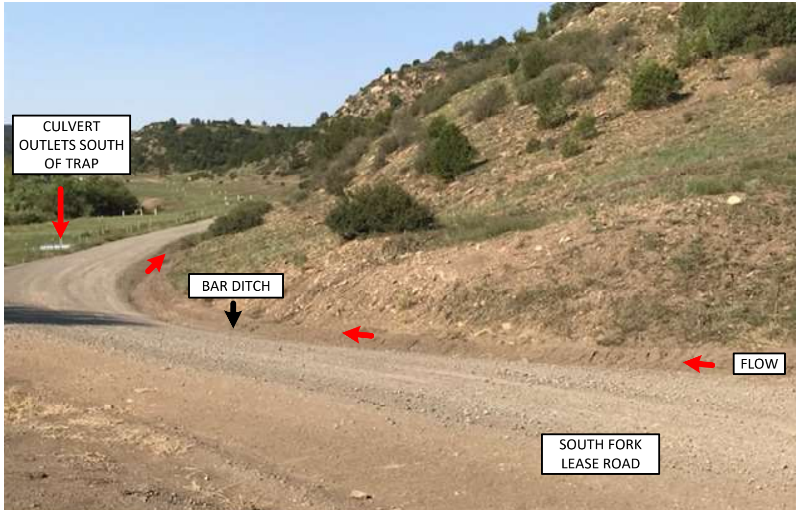
PHOTO 6: OVERFLOW FROM THE SEDIMENT TRAP IS DIRECTED TO THE CULVERT INLET DOWN GRADIENT OF THE SEDIMENT TRAP.
