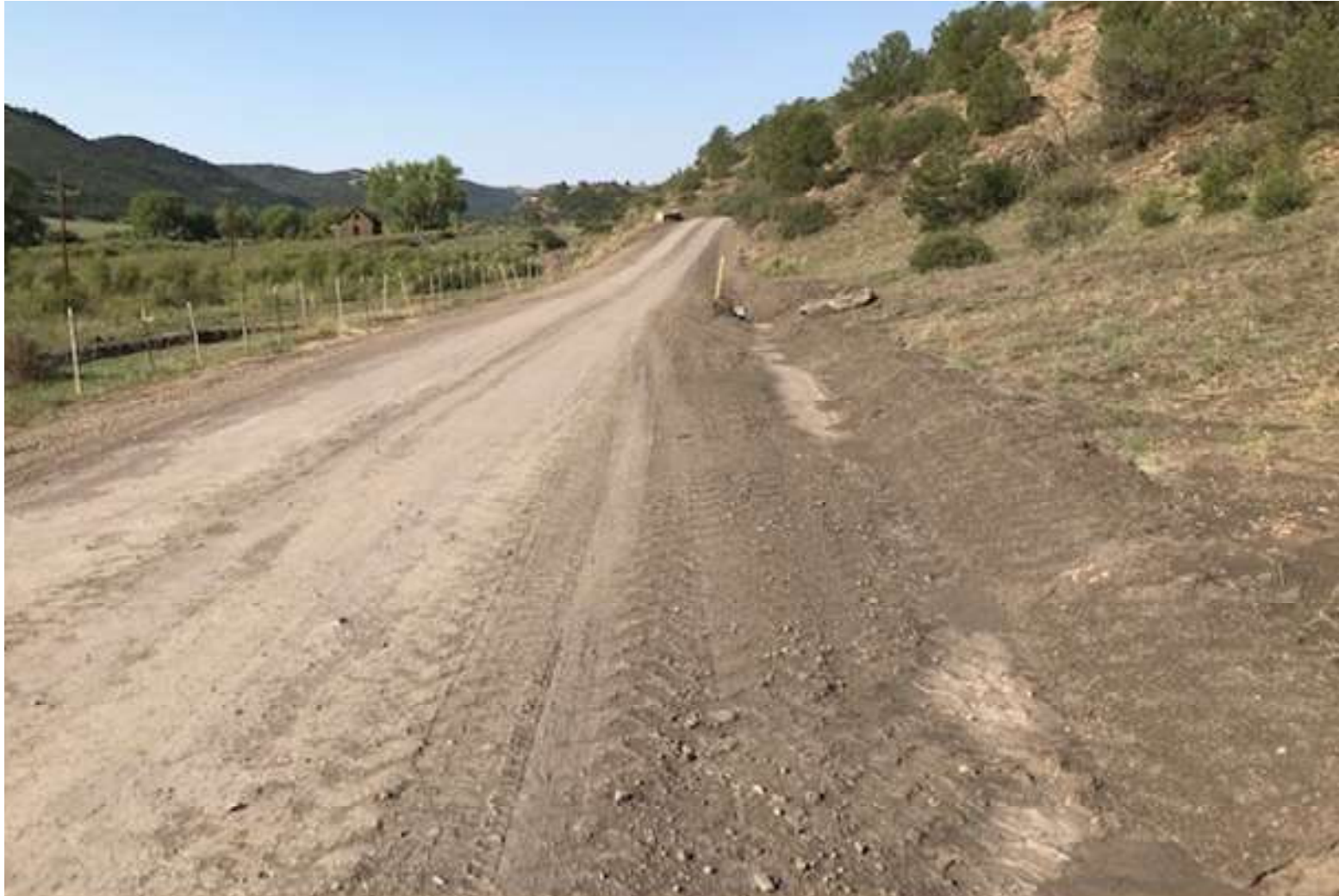
PHOTO 1: FACING SOUTHWEST ALONG THE MAIN ROAD IN SOUTH FORK. A NEW 36 INCH CULVERT WAS INSTALLED AND THE ROADWAY SURFACE REGRADED TO DIRECT STORMWATER RUNOFF TO THE CULVERT INLET.
