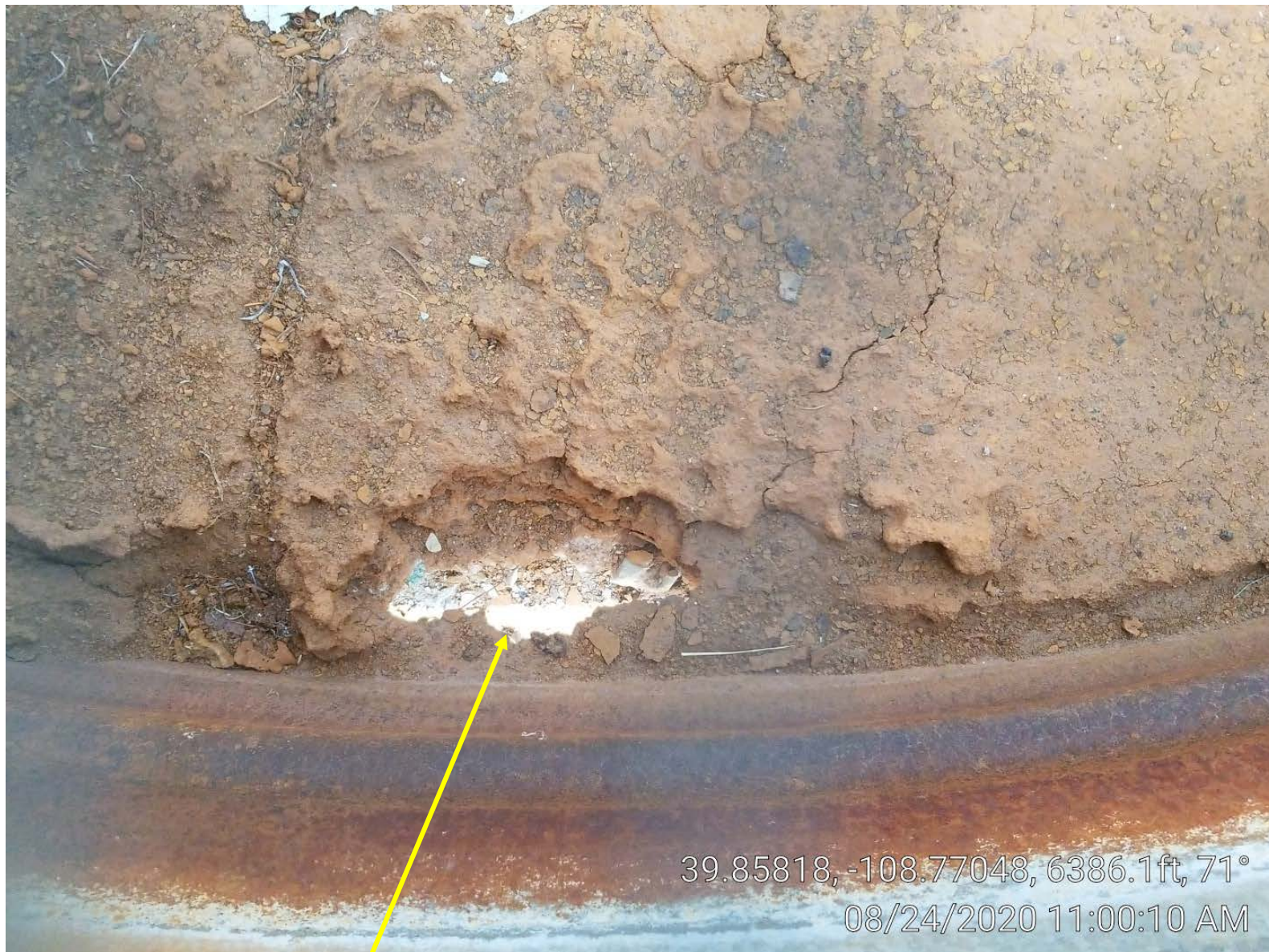
Photo 4. Hole in tank viewed from inside tank.
