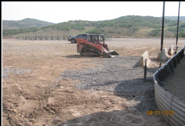
Road Base Installation on Pad 4A
