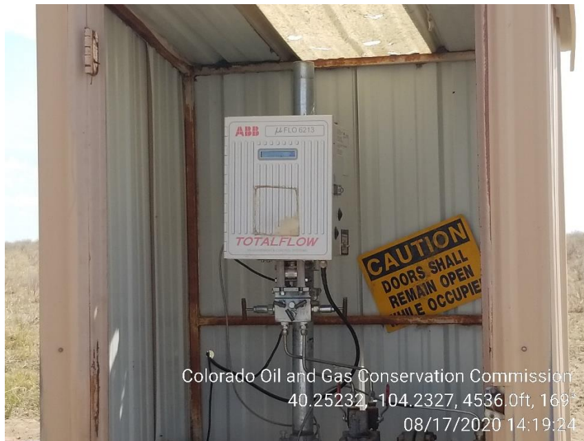
Photo 3 – Gas Meter appears to not be updated on Calibration.
