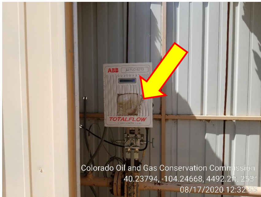
Photo 3 – Gas Meter, No Current Calibration card
