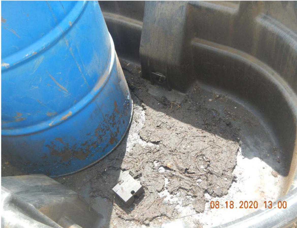
Photo #5 Close up of lube oil in secondary containment.
