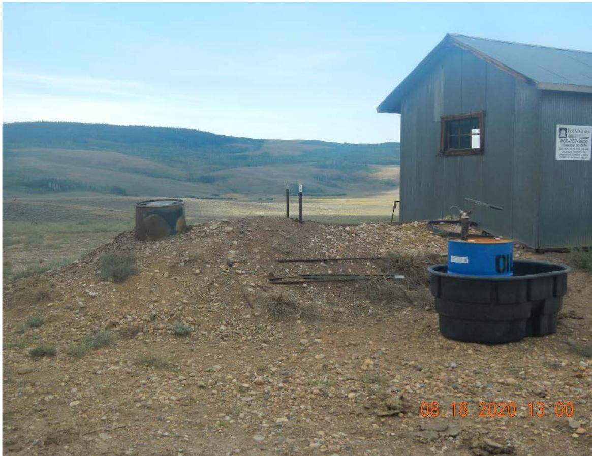
Photo #3 Motor shed for Pumpjack on right of photo. Barrel on left is a muffler for gas motor. Lube oil to right of photo in secondary containment.
