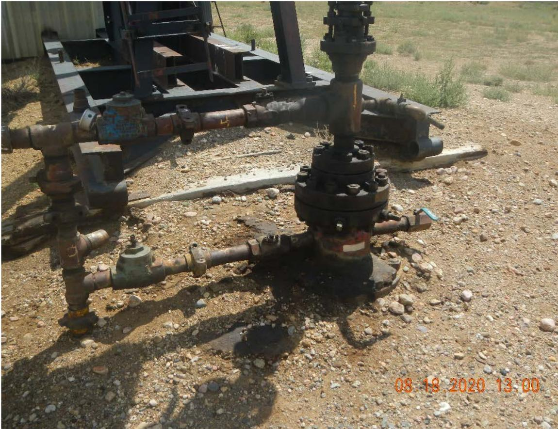
Photo #7 Wellhead. Some oil staining.
