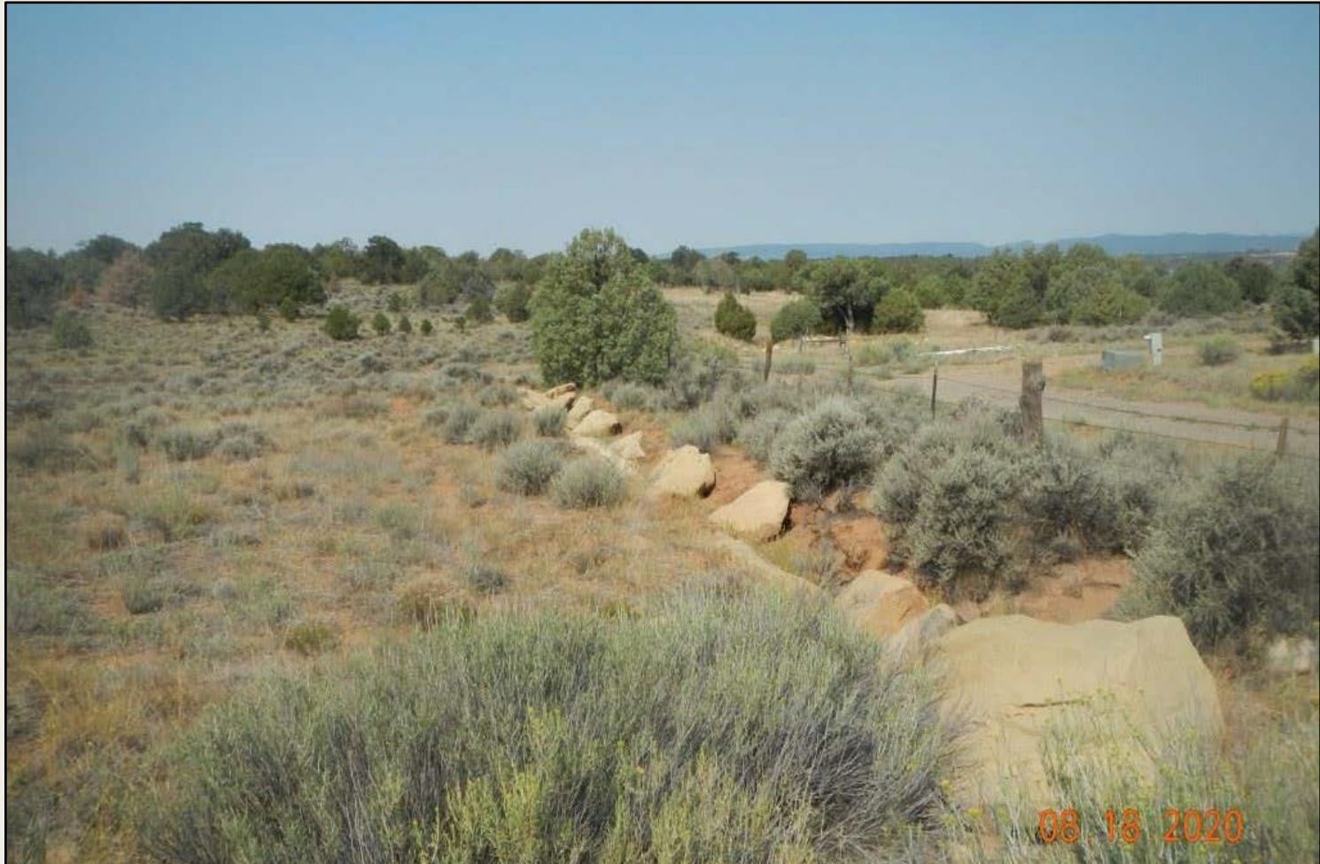
Photo 3. View of stormwater diversion northwest of the project area with boulders in place. Stormwater erosion appears to be controlled at this time.
