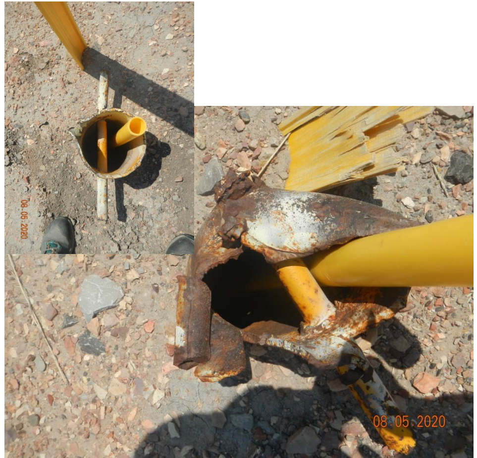
Photo#9: Other open pipe/risers that should be capped/filled.
