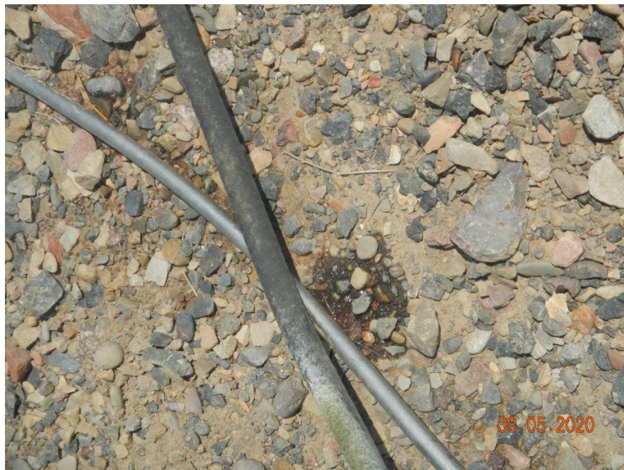
Photo#7: Drip from process pipe.
