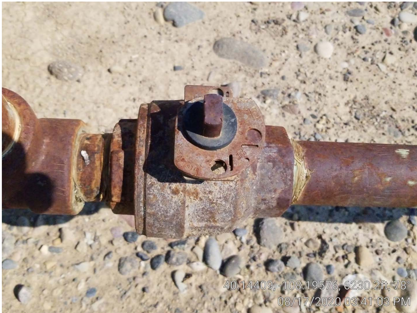
Photo 3. Casing valve.
