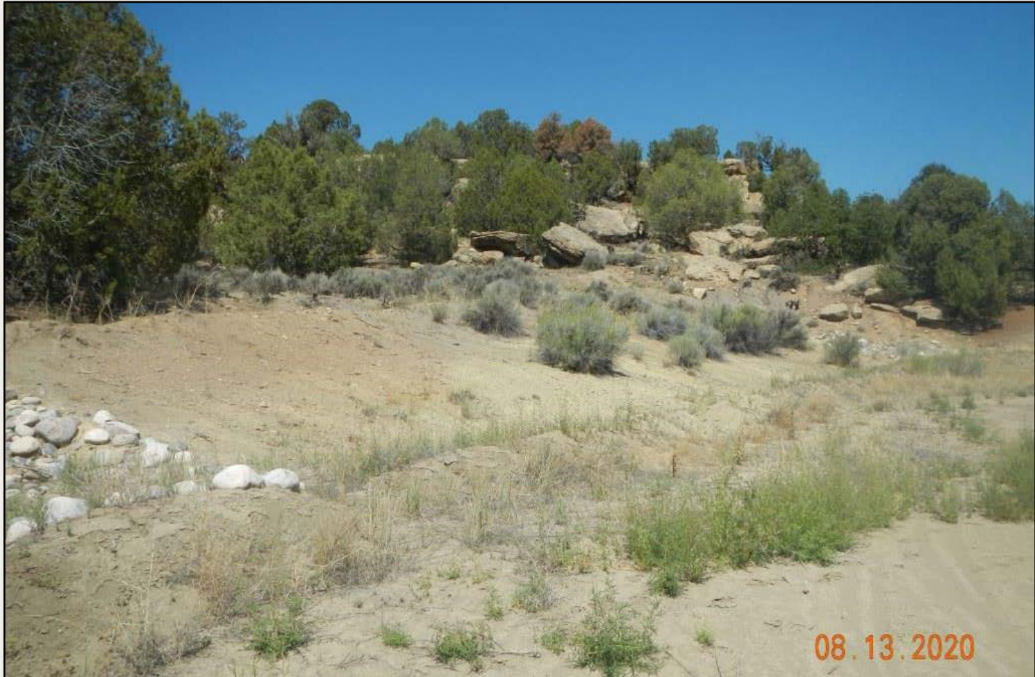
Photo 4. View of the western cut-slope facing northward. Berm is installed and seeded since 2017 reclamation inspection, diversion channel above slope, and cobble run-down. BMPs appear to be functioning. Monitoring needs to continue on slopes where bare soils persist.
