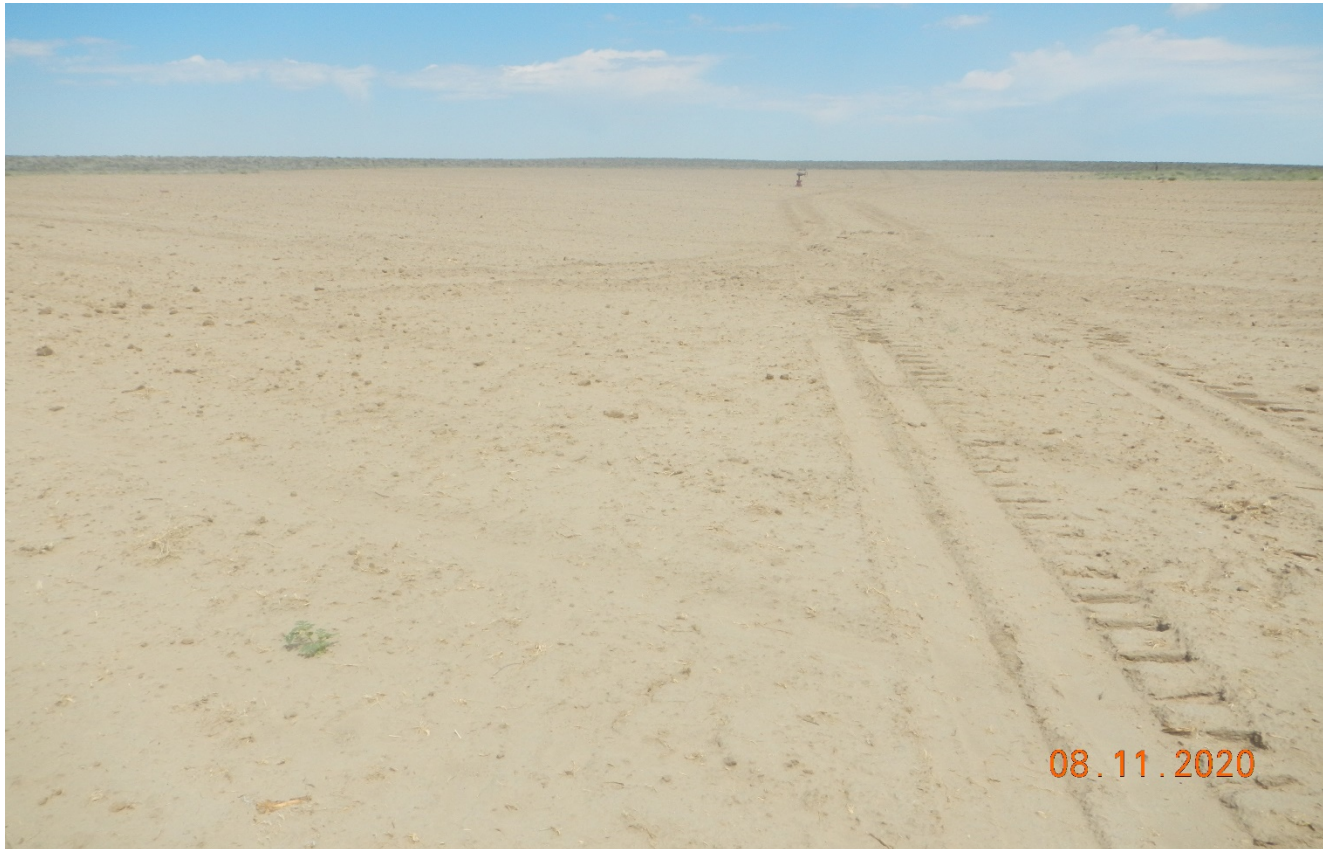
Photo 2. The pit has been backfilled and soil piles have been recontoured.
