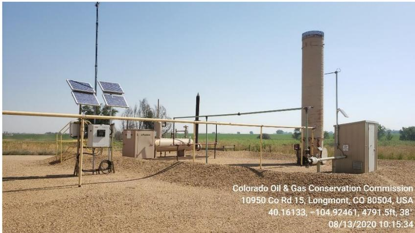
**Photo 9 Solar automation, Horiz. Heated Sep, ECD, and Gas Meter Run.**
